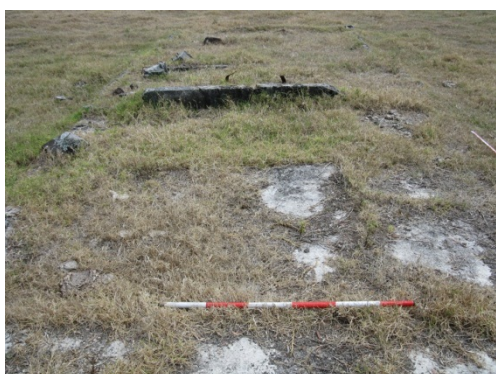
Figure E-23: Concrete foundations, facing west.
