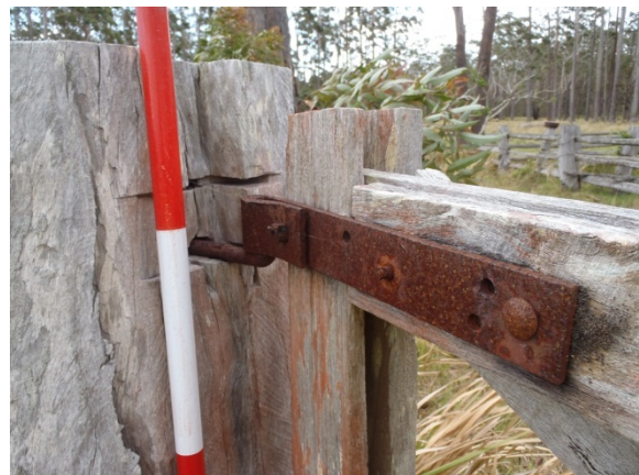
Figure E-4: Close up of metal hinge on gate.
