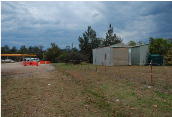
Figure E-6: Former Halfway Creek fire station and surrounds, facing south-east.
