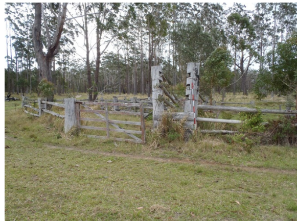
Figure E-2: Stockyards, facing north-west.
