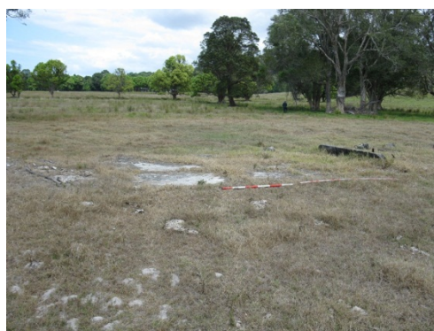
Figure E-24: Concrete foundations, facing south-west.
