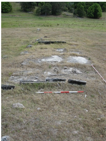
Figure E-21: Concrete foundations, facing west.
