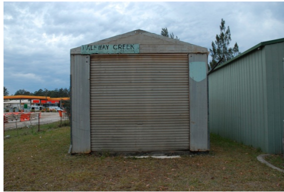
Figure E-7: Former Halfway Creek fire station, showing painted sign above roller door, facing south.
