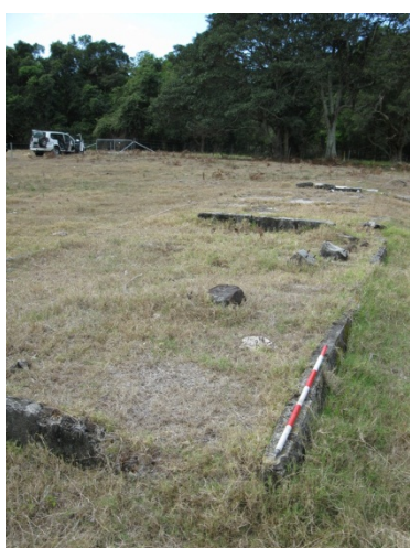
Figure E-25: Concrete foundations, facing north-east.
