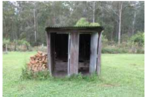
Figure 7-18: The outhouses, facing east-north-east, photo taken by Rachael Loizou on 28 October 2011.
