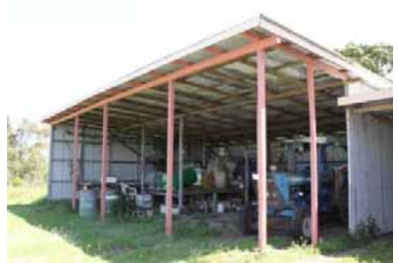
Figure 7-109: Open bay shed, facing south-west, photo taken by Rachael Loizou on 31 October 2011.
