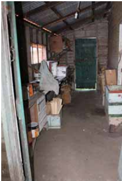
Figure 7-102: Interior of enclosed barn section of dairy, facing east, photo taken by Rachael Loizou on 31 October 2011.
