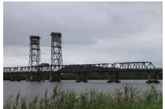
Figure 7-55: Harwood Bridge, facing south-east, photo taken by Rachael Loizou on 28 October 2011.
