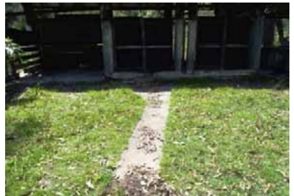
Figure 7-92: Western exterior side of main structure, facing east, photo taken by Rachael Loizou on 25 October 2011.
