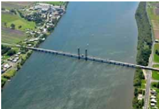
Figure 7-54: Harwood Bridge, facing east, photo taken for upgrade project aerial survey.
