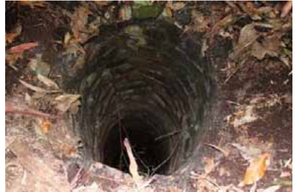
Figure 7-120: Brick lined well, facing south, photo taken by Rachael Loizou on 1 November 2011.
