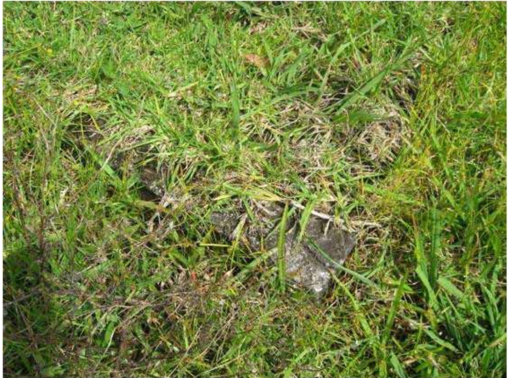
Figure 7-142: Rectangular concrete building foundations, photo taken by Joseph Brooke in November 2010.
