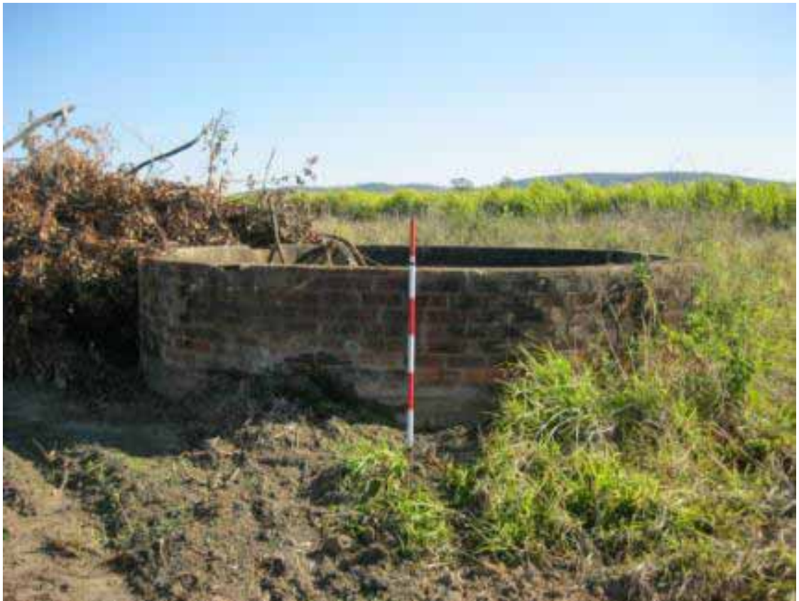
Figure 7-62: Concrete-lined brick well at property 315, photo taken by Vanessa Edmonds in August 2010.
