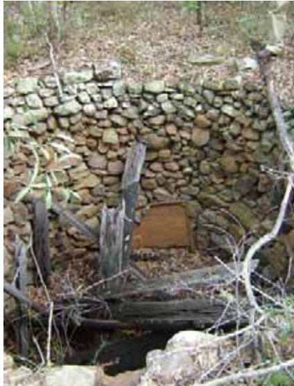
Figure 7-79: Roder's stone-lined well, photo courtesy of Richmond Valley Council, taken 2005.
