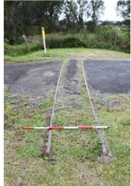
Figure 7-44: Old Pacific Highway Tram Tracks, facing east, photo taken by Rachael Loizou on 28 October 2011.
