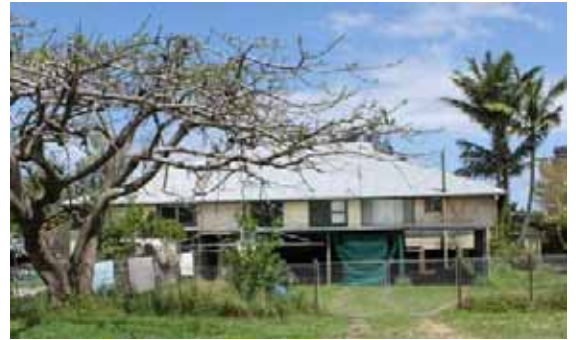
Figure 7-60: Rear of convent building, facing south, photo taken by Rachael Loizou on 31 October 2011.
