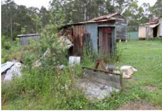
Figure 7-19: Shed 2, facing south-south-west, photo taken by Rachael Loizou on 28 October 2011.
