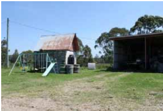
Figure 7-110: Buttery/creamery, facing south-west, photo taken by Rachael Loizou on 31 October 2011.
