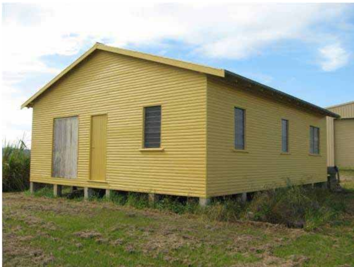
Figure 7-31: Tyndale Cane Barracks, photo taken by Joseph Brooke in November 2010.
