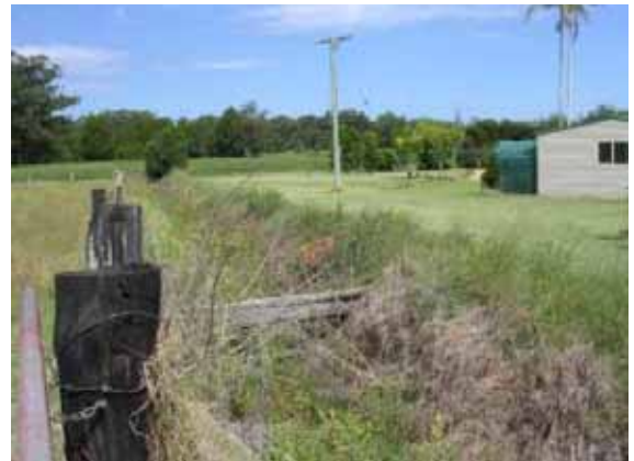
Figure 7-138: Drainage Union drainage channel (Heritage Concepts 2005).
