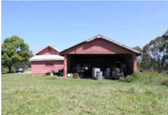
Figure 7-100: Dairy with open timber barn at right and enclosed timber barn section at left, facing south, photo taken by Rachael Loizou on 31 October 2011.
