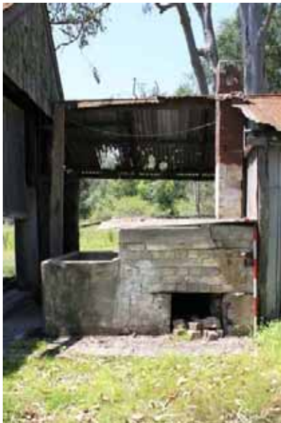
Figure 7-95: Copper, fuel box, chimney and trough, facing east, photo taken by Rachael Loizou on 25 October 2011.
