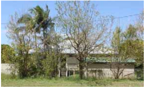
Figure 7-59: West side of convent building, facing east, photo taken by Rachael Loizou on 31 October 2011.
