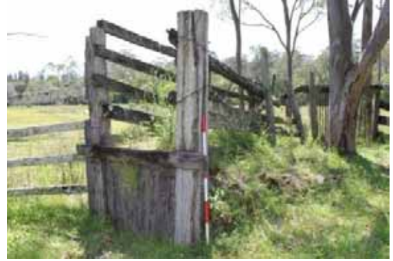
Figure 7-98: Cattle ramp, facing north, photo taken by Rachael Loizou on 25 October 2011.
