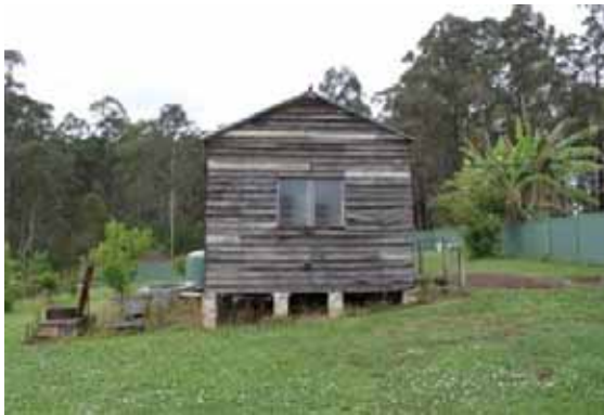
Figure 7-17: Shed 1, facing south, photo taken by Rachael Loizou on 28 October 2011.
