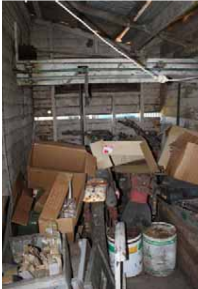
Figure 7-104: Interior of enclosed barn section of dairy showing milk pipeline, facing south, photo taken by Rachael Loizou on 31 October 2011.
