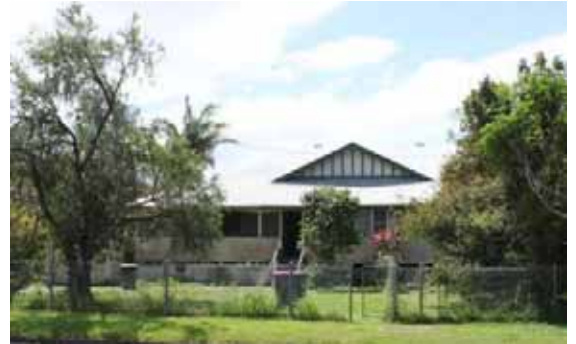
Figure 7-58: Front of convent building, facing north, photo taken by Rachael Loizou on 31 October 2011.
