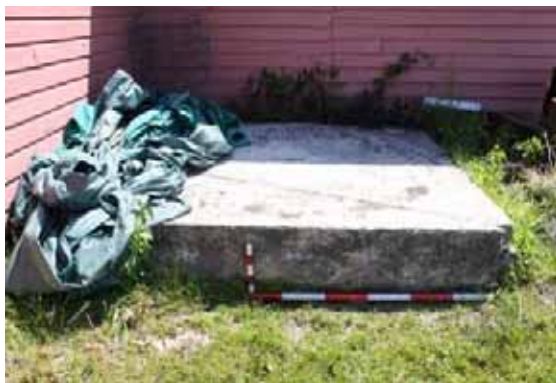
Figure 7-106: Concrete block, facing west, taken by Rachael Loizou on 31 October 2011.
