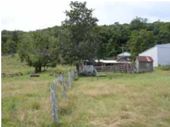
Figure 7-137: Original dairy buildings (Heritage Concepts 2005).
