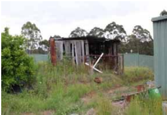
Figure 7-21: Shed 3, facing west-south-west, photo taken by Rachael Loizou on 28 October 2011.
