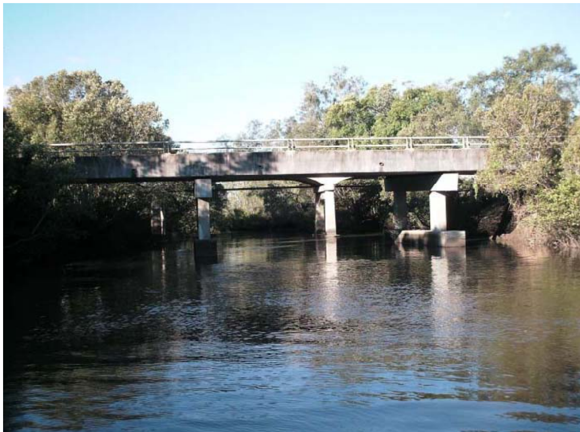
Plate 4-16 Serpentine Channel looking upstream
