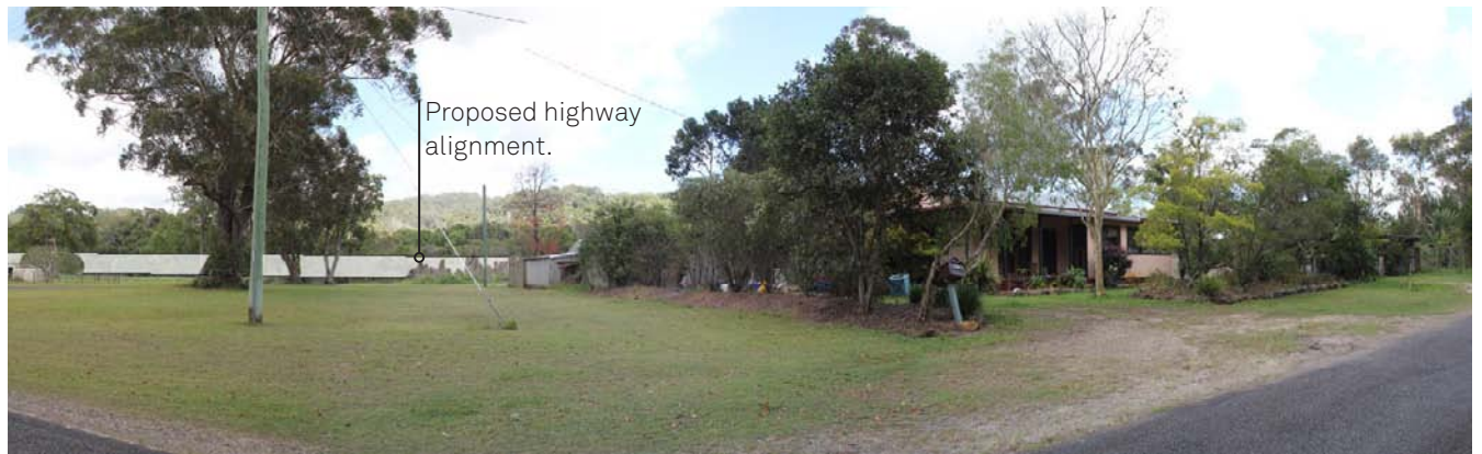
Annotated diagrammatic approximation of the project as photographed from viewpoint 58_ View west, Pimlico Road, Pimlico. Location: 28°55'10"S 153°28'41"E
