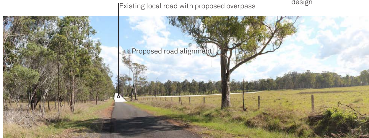
Annotated diagrammatic approximation of the project as photographed from viewpoint 10_ View south, Avenue Road. Location: 29°44'58"S 153°03'52"E.
