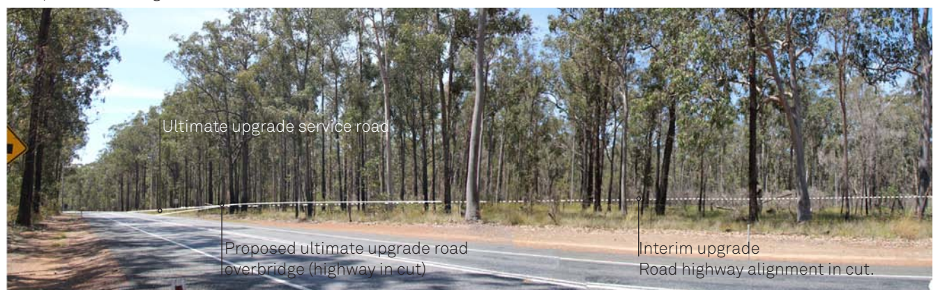
Annotated diagrammatic approximation of the project as photographed from viewpoint 4_ View north east, Pacific highway, south of Bald Knob Tick Gate Road. Location: 29°52'39"S 153°03'27"E.
