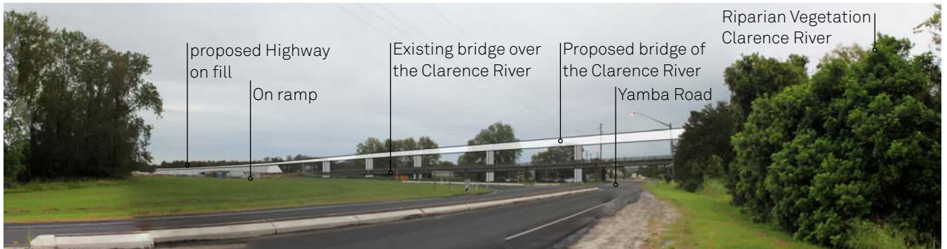
Annotated diagrammatic approximation of the project as photographed from viewpoint 26B_ View west along Yamba Road, Harwood (South). Location: 29°25'58"S 153°14'31"E
