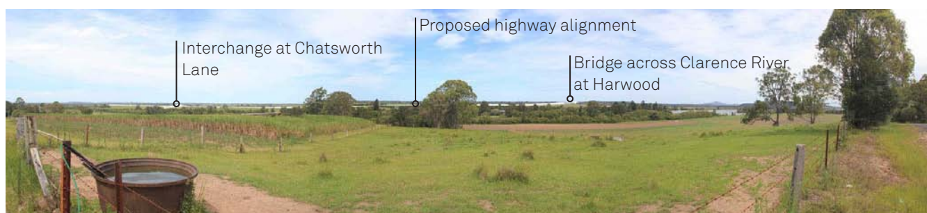
Annotated diagrammatic representation of the project as photographed from viewpoint 31_ Murrayville Road, Ashby Heights. Location: 29°24'21"S 153°12'34"E
