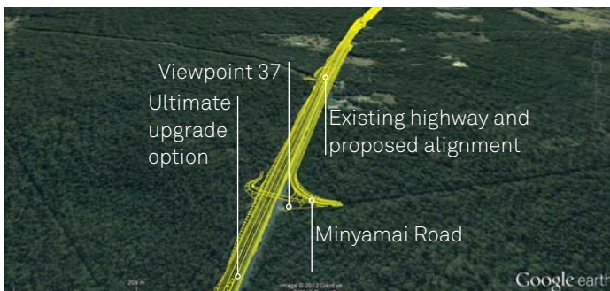
Oblique view looking north
