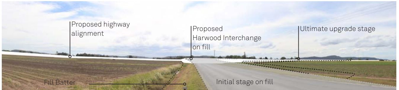
Annotated diagrammatic approximation of the project as photographed from viewpoint 32_ Watts Lane (East), Harwood. Location: 29°25'09" S 153°14'35" E
