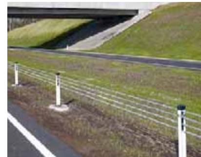
Frangible median vegetation will reduce headlight glare.
