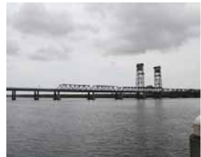
Existing Harwood Bridge to be retained as a significant place marker along the journey. HASSELL image
