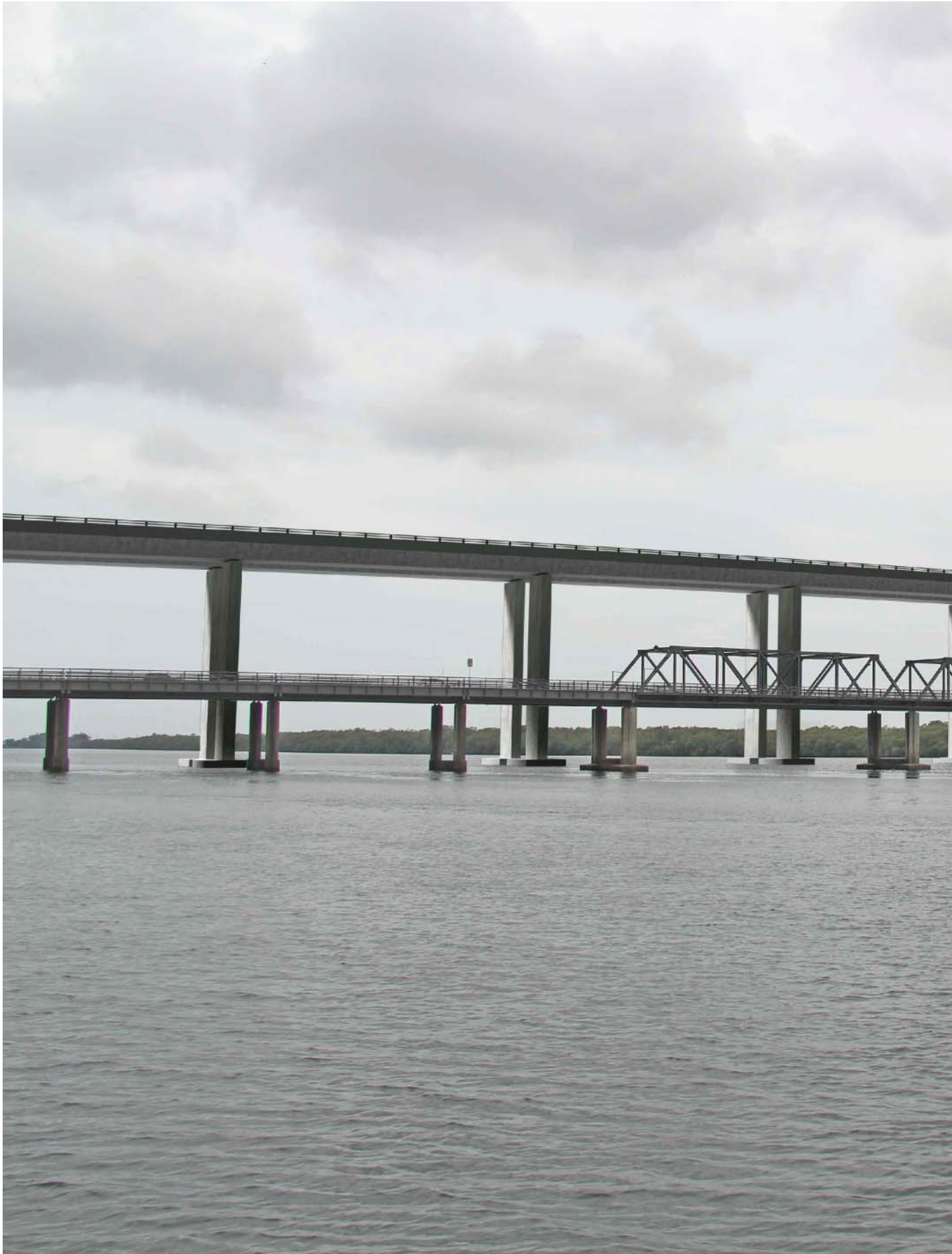
Ground view of the bridge crossing the Clarence River at Harwood, looking south east . Box girder bridge design
