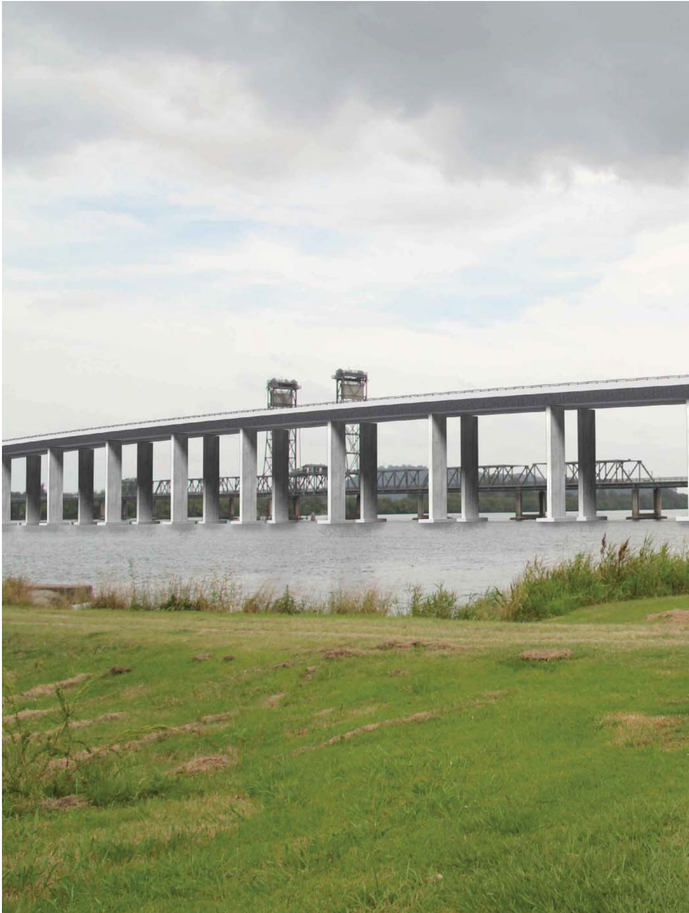
Ground view of the bridge crossing the Clarence River at Harwood, looking south west Box girder bridge design
