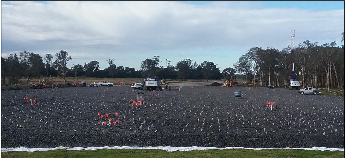
Soft soil work – foundation rock being placed north of Tuckombil Canal, August 2016
