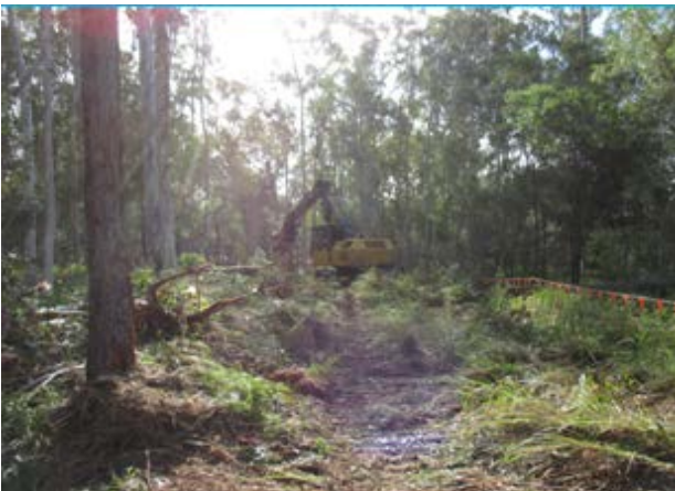
Clearing work underway near Lemon Tree Road at Halfway Creek
