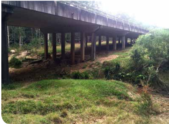
Tabbimobile creek old bridge before rehabilitation May 2016
