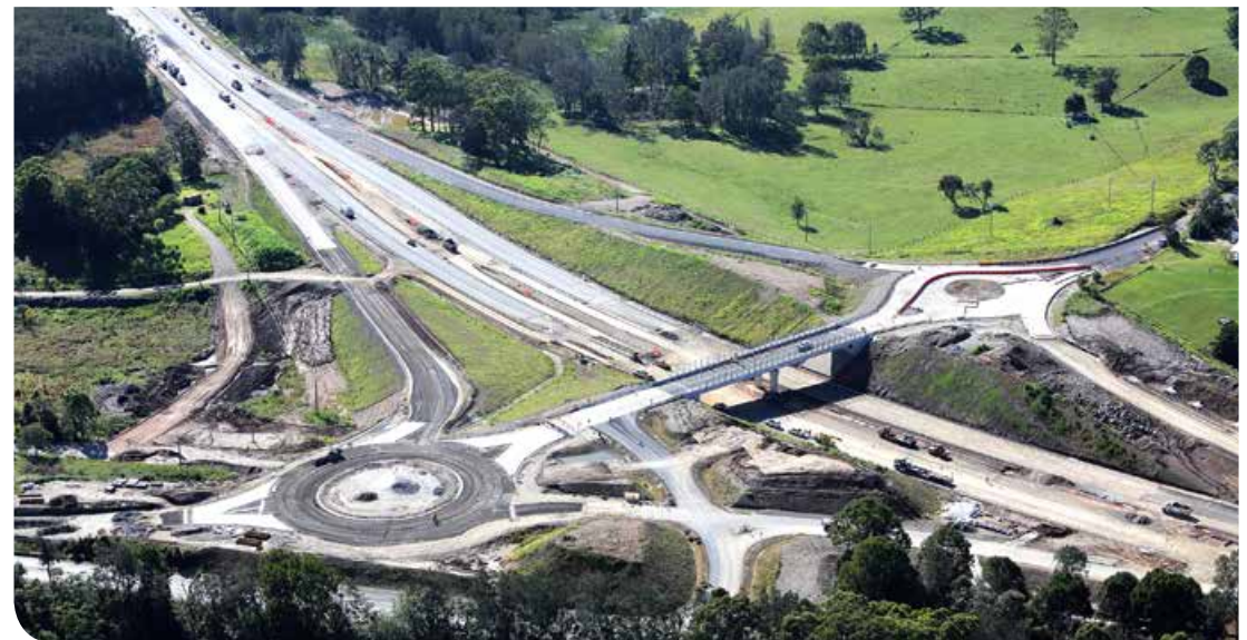
Bald Hill Road interchange looking south (June 2017)
