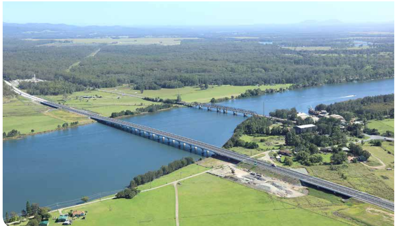
Aerial view of the new bridge over the Hastings River looking north east, December 2017
