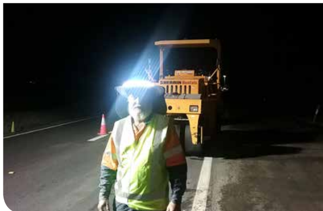
A worker trials the halo light during night work at Broadwater
