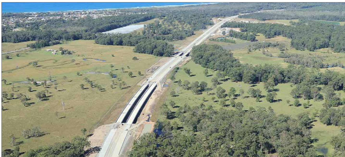
Aerial view of the new bridges over the floodplain near Corindi Beach
