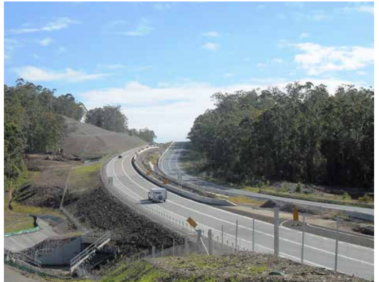
New northbound lanes near Dirty Creek
