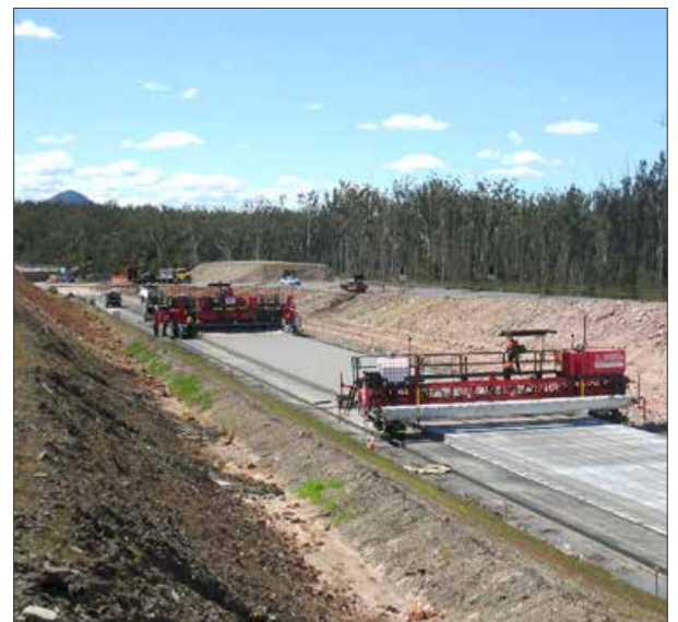
Paving on northbound carriageway south of Wells Crossing
