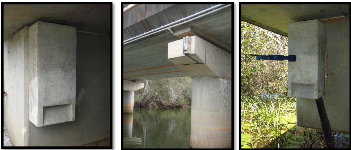
Plate 4-2. Bat boxes installed at a low culvert structure at Urunga (left and right) and Deep Creek, Valla (middle) using the full height capacity of each structure.
