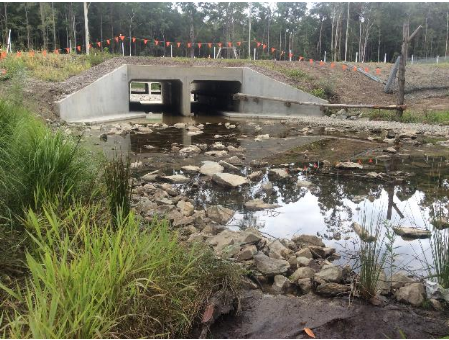
Fauna underpass with internal and external fauna furniture installed
