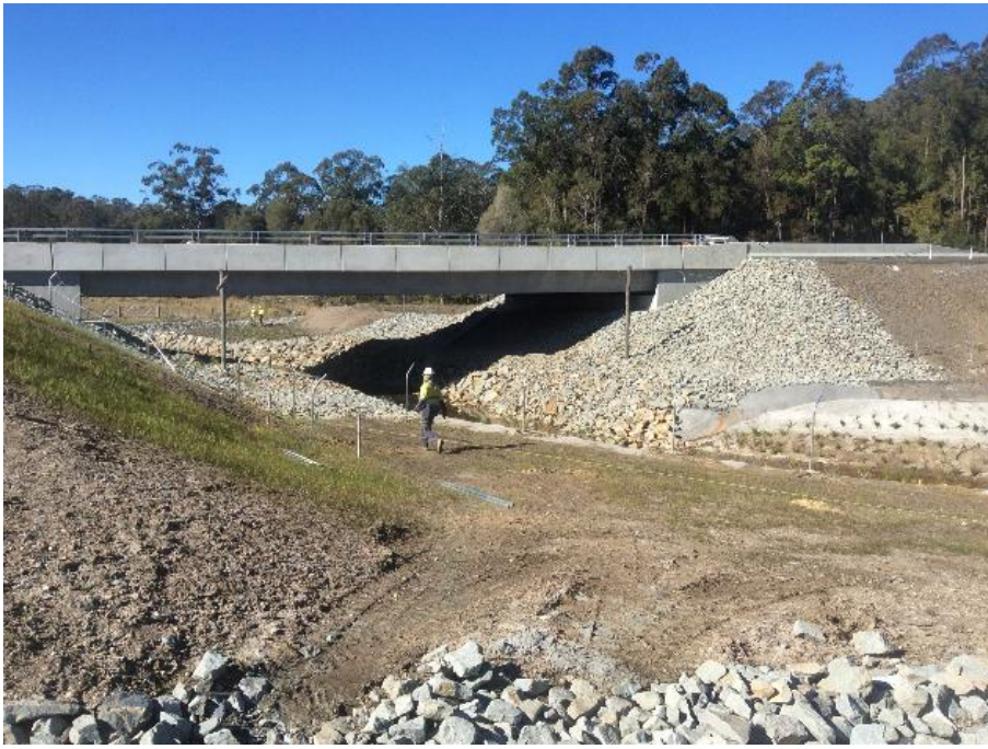
Fauna exclusion fencing being completed at SB20 fauna underpas
