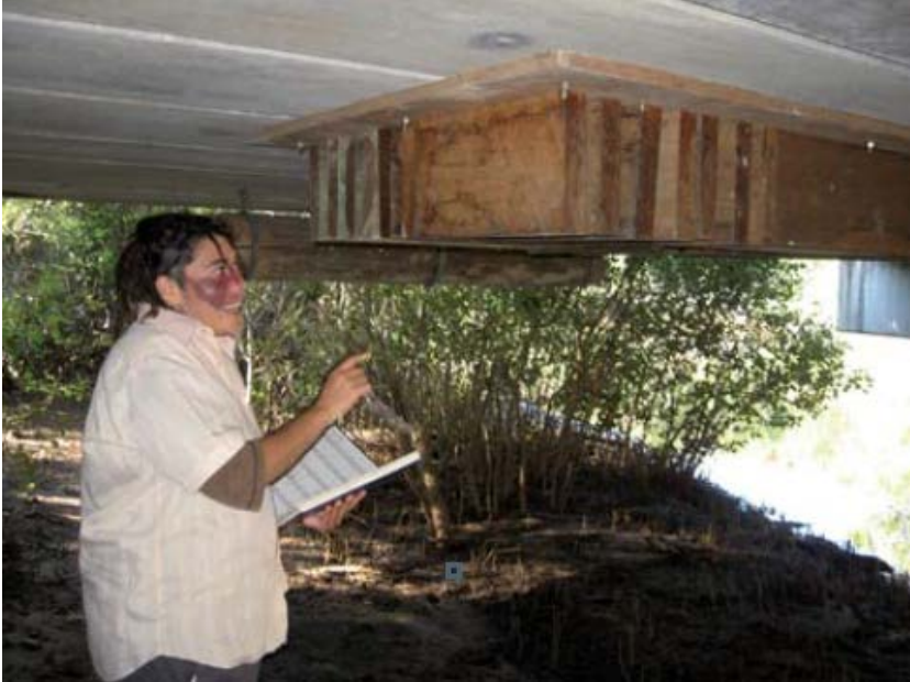
Plate 1: Artificial roost for Myotis macropus under bridge at Kioloa Beach NSW. Photo from Marshall (2011).
