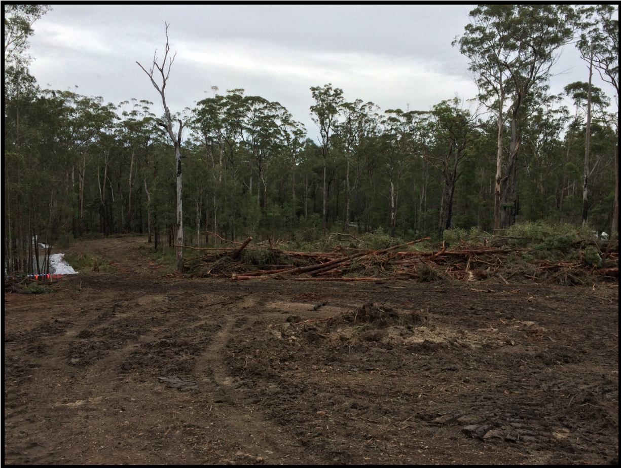
Plate 3-4. Clearing operations at the time of the unexpected Stephens Banded Snake find.
