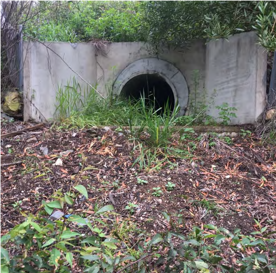
Plate 3: Habitat surrounding south-east frog pipe. (Picture taken 6 July 2017).
