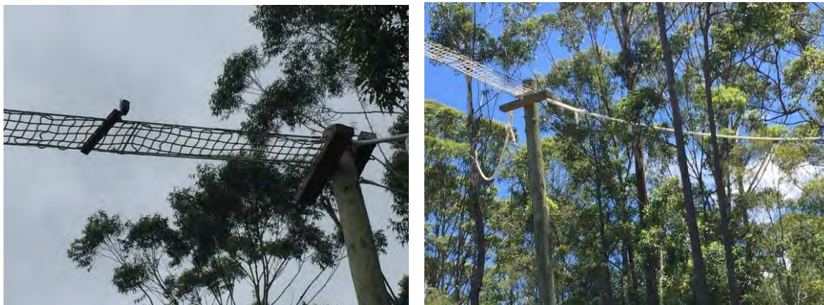
Plate 16: A Reconyx camera mounted to a wooden ‘sandwich board’ was positioned approximately 2m from each end of the rope bridge to capture moving fauna (left). Slung rope (25mm diam.) was used to link the bulkhead to surrounding trees (right).
