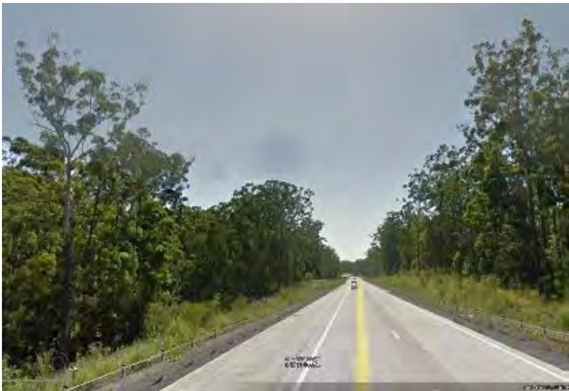
Plate 6: Vegetated median and adjoining habitat at Arrawarra (ch.29100-30200) as viewed along the east/southbound (top) and west/northbound (bottom) side of the alignment. The vegetated median is on the right side of both images. (Image: Google Earth).
