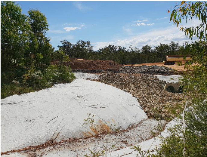
Photograph 10: Year 2 construction in-situ Site Li-3.1 showing cleared habitat and geofabric for drainage line and natural vegetation regeneration on edges (November 2018)
