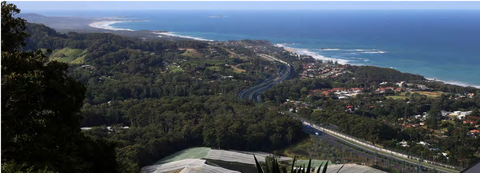
Figure 11-19 Viewpoint 20 showing the project with embedded mitigation
