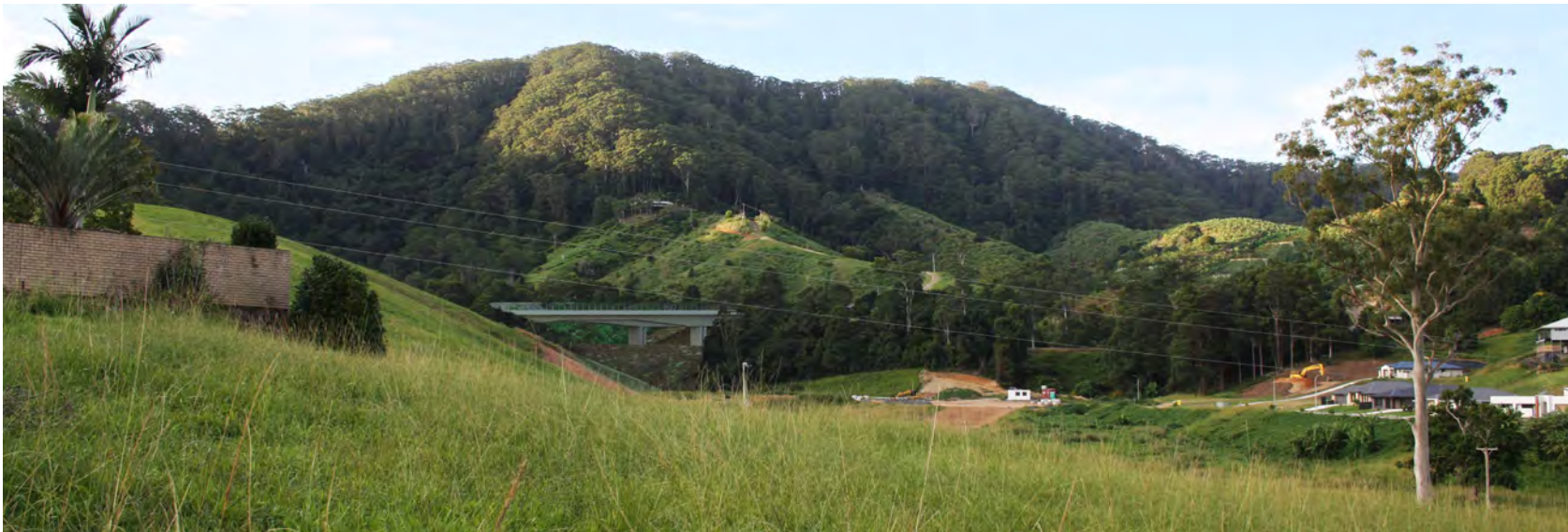
Figure 11-13 Viewpoint 11 showing the project with embedded mitigation
