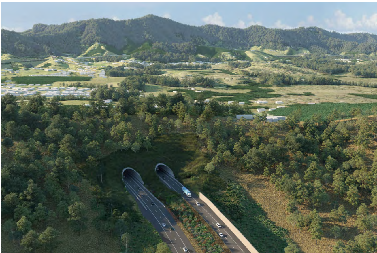
Figure 11-3 Roberts Hill tunnel
