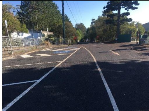
Korora School Road Car Park 7:40am (facing NB)
