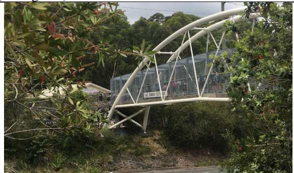
Students crossing Luke Bowen Footbridge at 3:20pm from eastern side of Pacific Highway
