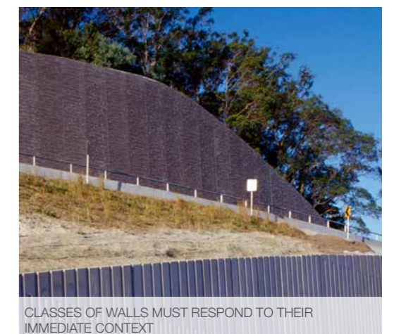
TOP EDGES OF THE RETAINING WALL TO PROVIDE A SMOOTH FLOWING ELEVATION (NO STEPPING)
