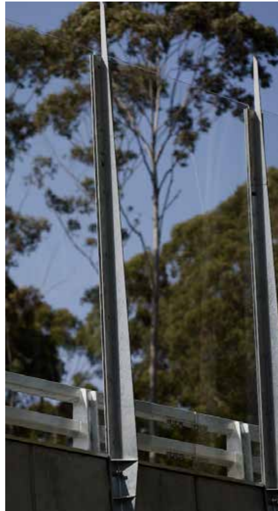
THE DESIGN SHOULD COMPRISE STEEL POSTS WITH TRANSPARENT PANELS.
