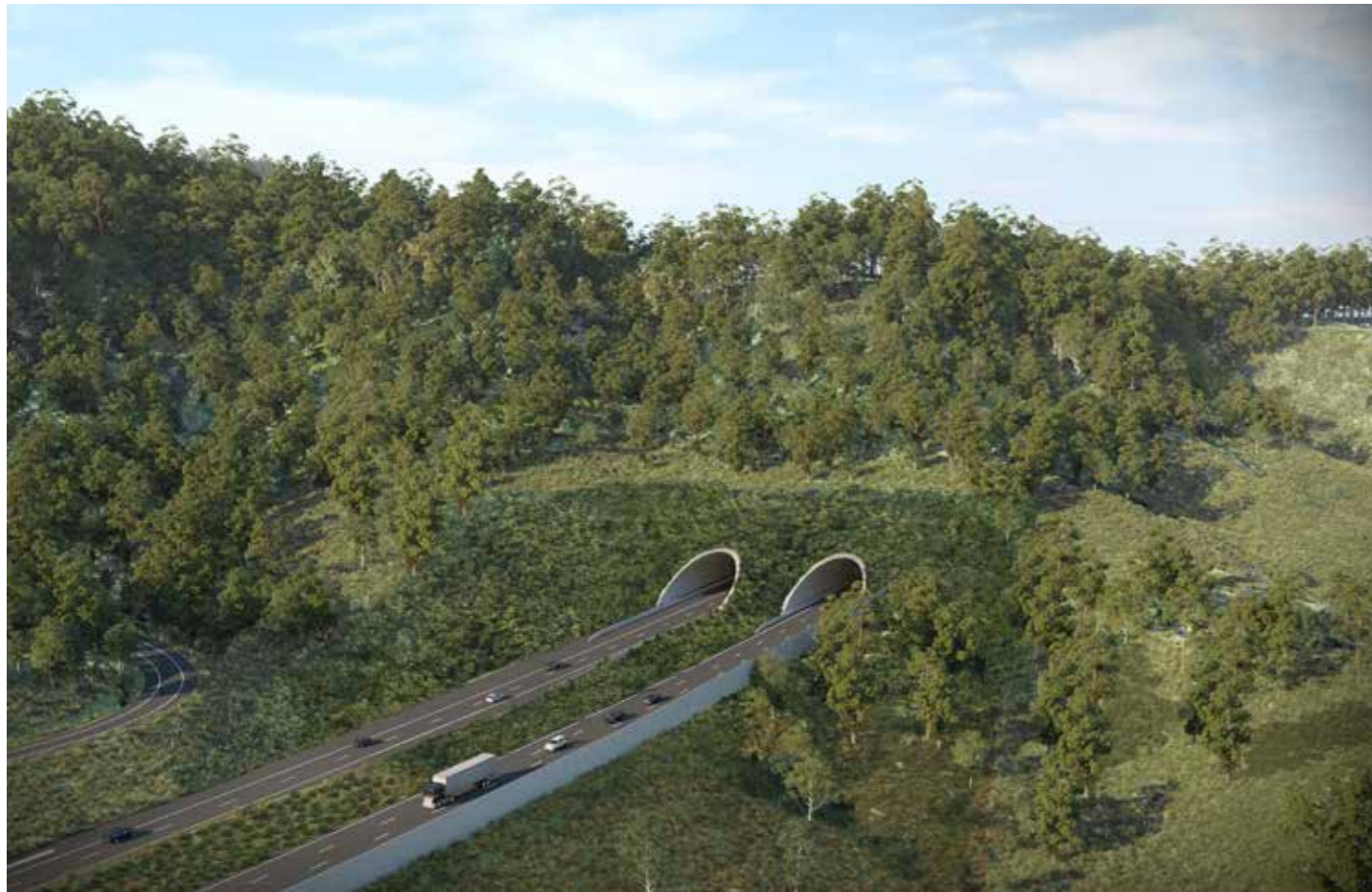
FIG 1.5 GATELYS ROAD TUNNEL - SOUTHERN PORTAL
