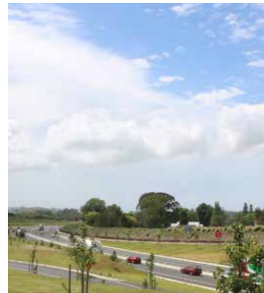
FILL EMBANKMENTS TO HAVE 2H:1V BATTERS OR FLATTER FOR STABILITY (PHOTO: BERRY BYPASS)
