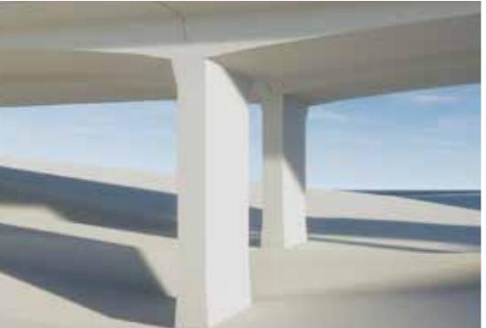
FIG 5.29 PIER OPTION 3 - CANDLESTICK
