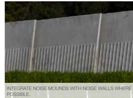
MINIMISE THE VISUAL IMPACT OF THE WALLS BY MINIMISING HEIGHT AND PROVIDE PLANTING TO SCREEN WALLS (SAPPHIRE TO WOOLGOOLGA)
