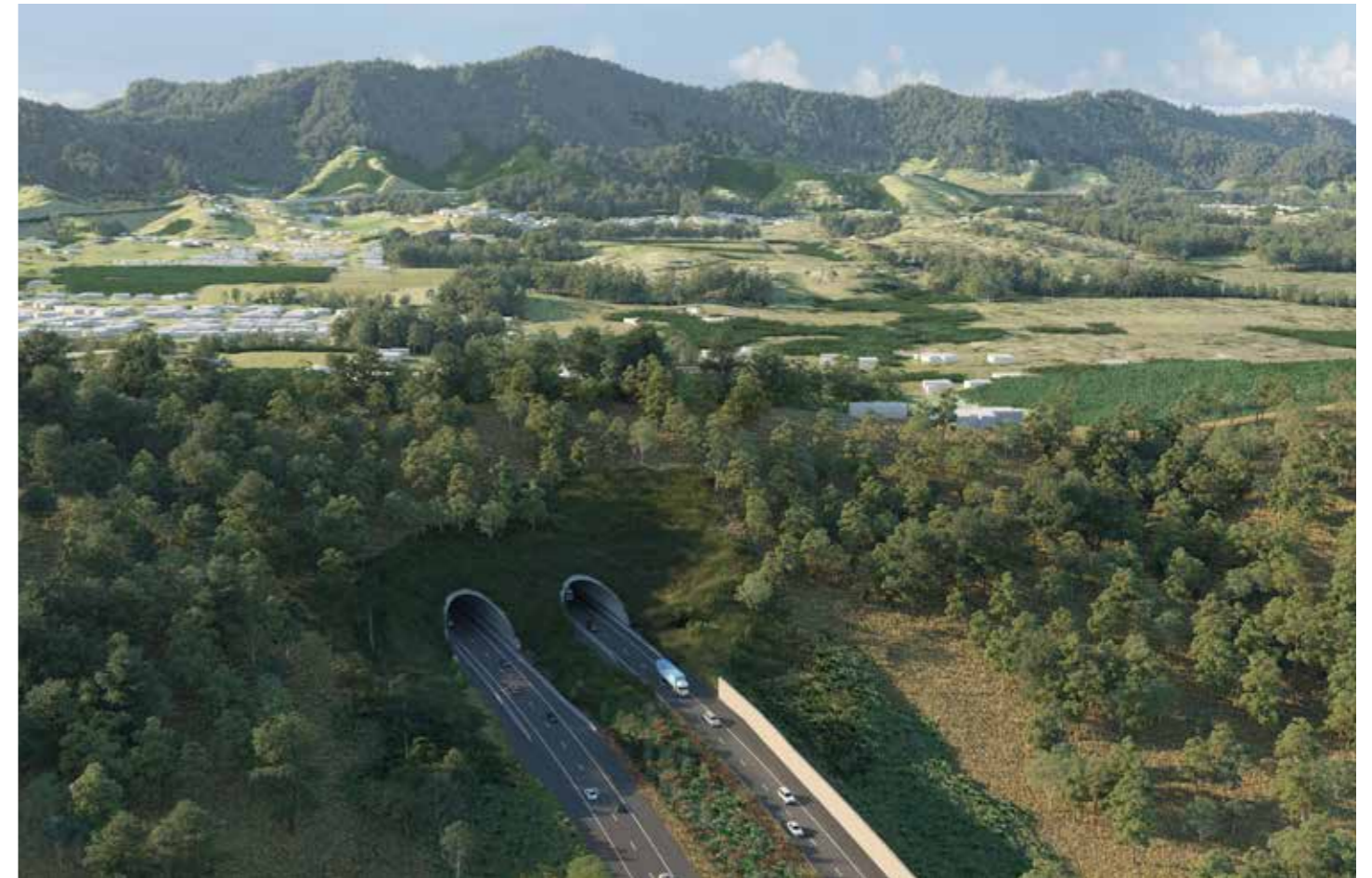
FIG 1.2 ROBERTS HILL TUNNEL - SOUTHERN PORTAL
