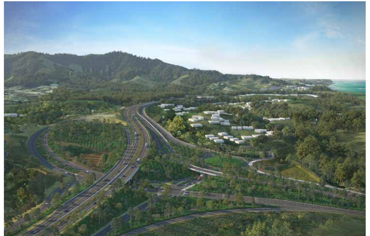
FIG 1.6 KORORA HILL INTERCHANGE
