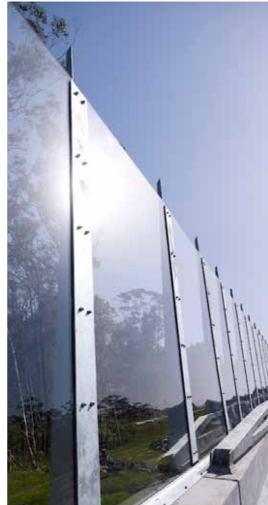
TRANSPARENT WALLS ENABLE VIEWS OUT FROM THE HIGHWAY TO THE SURROUNDING CONTEXT
