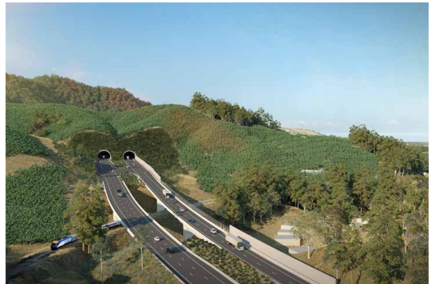
FIG 1.4 SHEPHARDS LANE TUNNEL - SOUTHERN PORTAL
