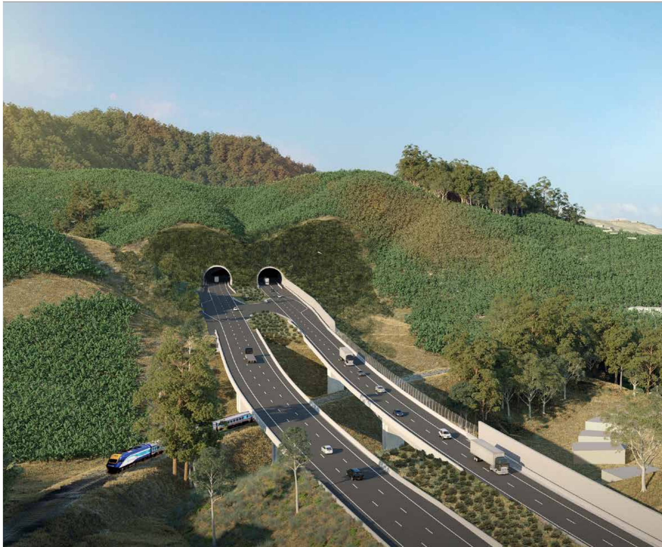
FIG 5.38 SHEPHERDS LANE TUNNEL - SOUTHERN PORTAL - CONCEPT DESIGN
