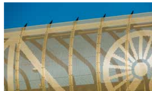
PERFORATED METAL SCREEN WITH INTERPRETIVE ART WORK AT HAWTHORNE STATION, SYDNEY LIGHT RAIL
