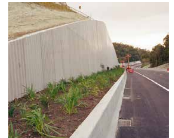
TOP EDGES OF THE RETAINING WALL TO PROVIDE A SMOOTH FLOWING ELEVATION (NO STEPPING)
