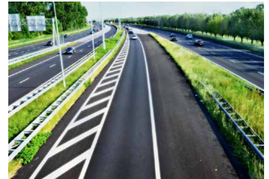
FIG A.2 PLANTING TO ALLOW FOR SURVEILLANCE, LOW PLANTING ADJACENT TO THE ROADWAY AND TREES WITH HIGHER CANOPY (CLEAR TRUNKS) LIMITING CONCEALMENT.
