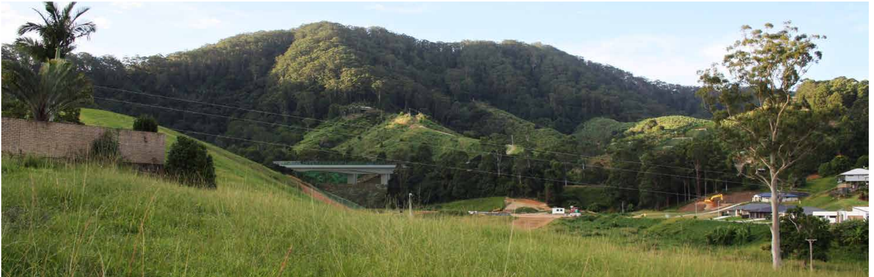
Viewpoint 11: Shephards Lane (embedded mitigation)
