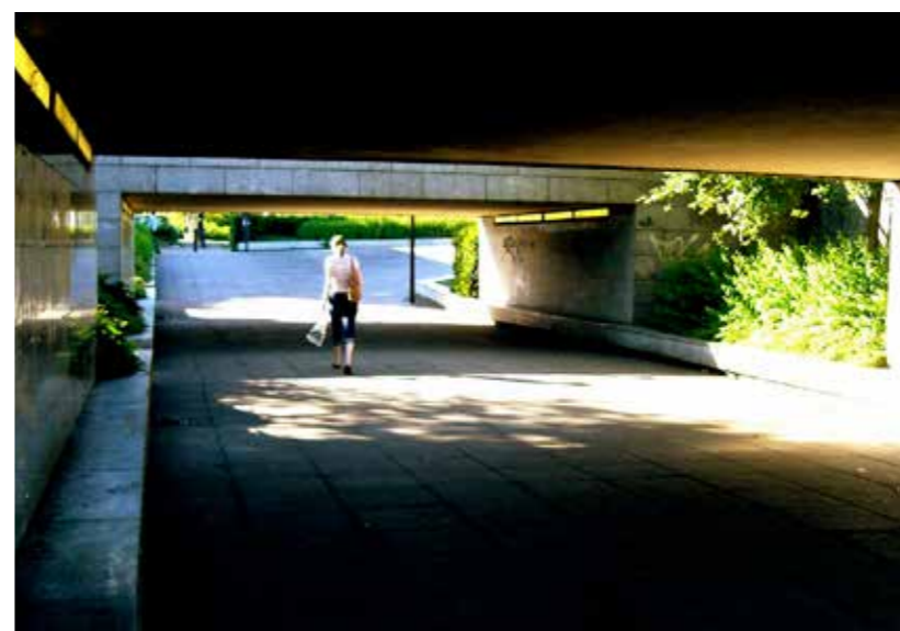
FIG A.3 WIDE PEDESTRIAN UNDERPASS. WHERE AN UNDERPASS NEEDS TO BE LONG, HAVING A DAY LIGHT OR OPEN SECTION HALF WAS IMPROVES THE USER EXPERIENCE.
