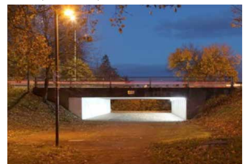
FIG A.4 UNDERPASS WITH CLEAR SIGHT LINES, UNOBSTRUCTED APPROACHES AND CLEARLY LIT UNDERNEATH.
