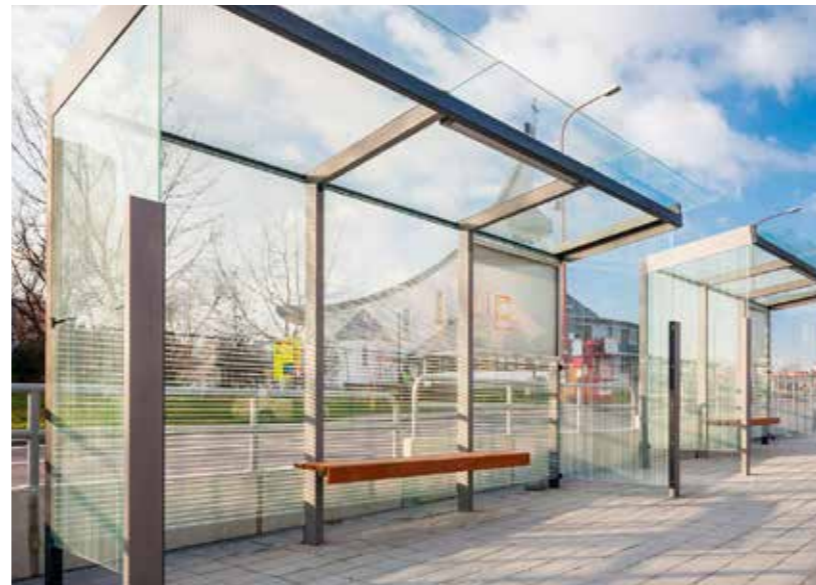
FIG A.13 AN EXAMPLE OF A BUS SHELTER WITH GOOD VISUAL PERMEABILITY AND FREE OF OBSTRUCTIONS.
