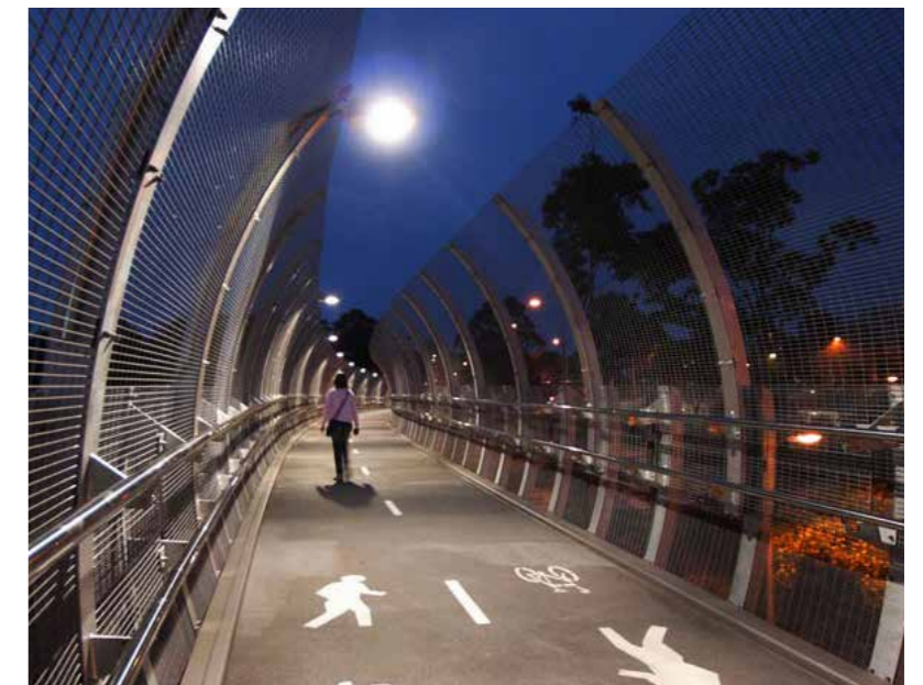
FIG A.12 A PEDESTRIAN BRIDGE WITH CLEAR SIGHT LINES ALONG THE LENGTH AND CLEARLY LIT.
