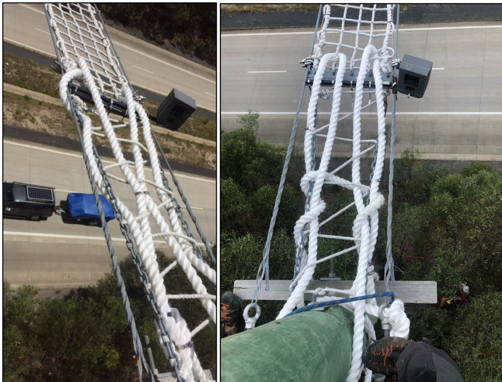
Plate 2.1 Silver rope addition at rope bridge chain on the eastern pole (left) and western pole (right)
