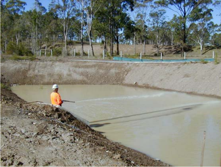
Figure 1. Application to a sediment basin allows faster settling of sediments and improvements to water quality prior to discharge.
