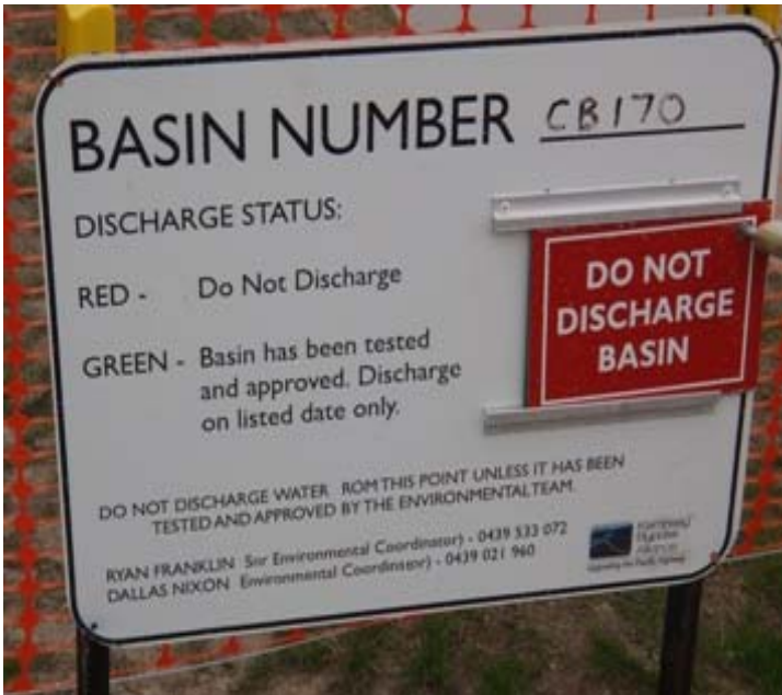
Figure 3. Use of formal signage indicating discharge procedures was an effective management tool to prevent unauthorised discharges.
