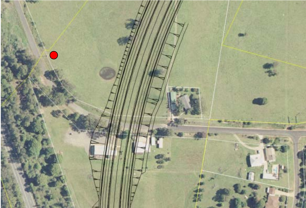
Plate 4.3 Monitoring Sites for Project Chainage 49,365 : Cut 12 (Type A high-risk cutting)
