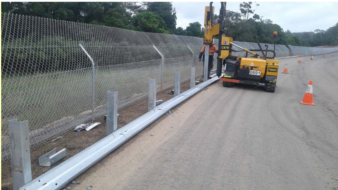
Photo 4: Finishing Works prior to opening - Fauna Fencing and guardrail installation
