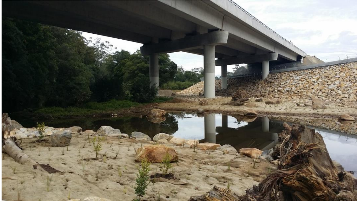
Photo 5: Upper Warrell Creek – restoration of Giant Barred Frog Habitat
