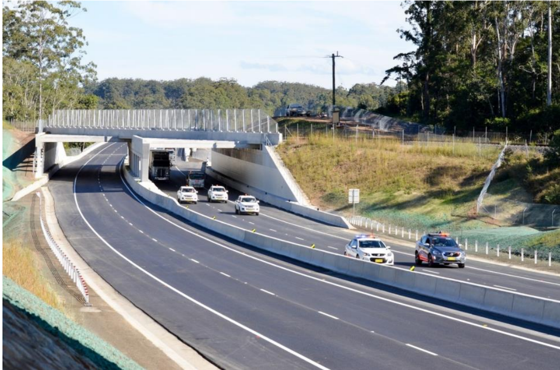
Photo 1: Opening of Stage 2B (Full Opening) – north bound traffic escorted by police under the ARTC railway at Upper Warrell Creek
