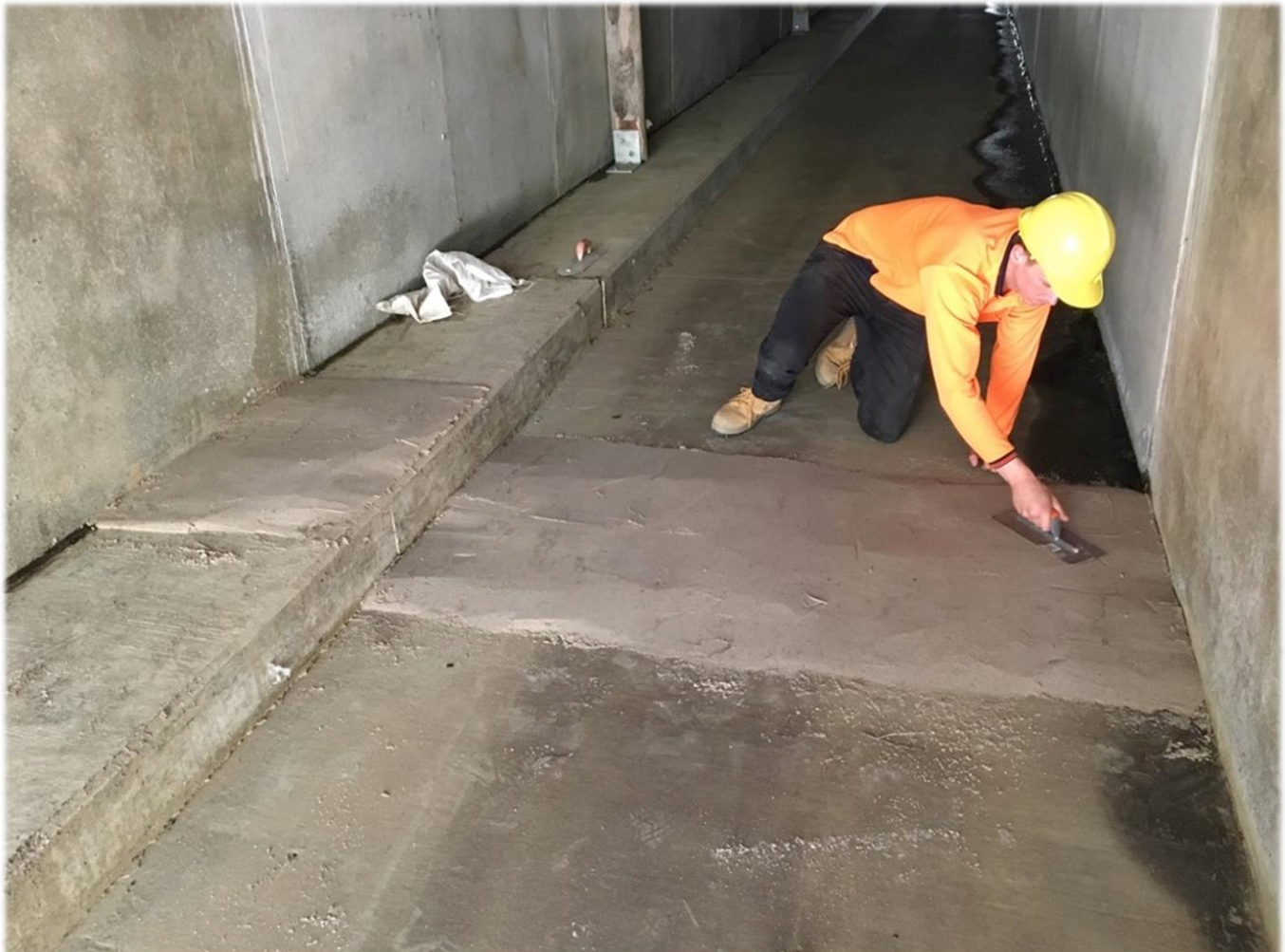
Plate 1: Sand pad being installed in a fauna underpass on the WC2NH upgrade.
