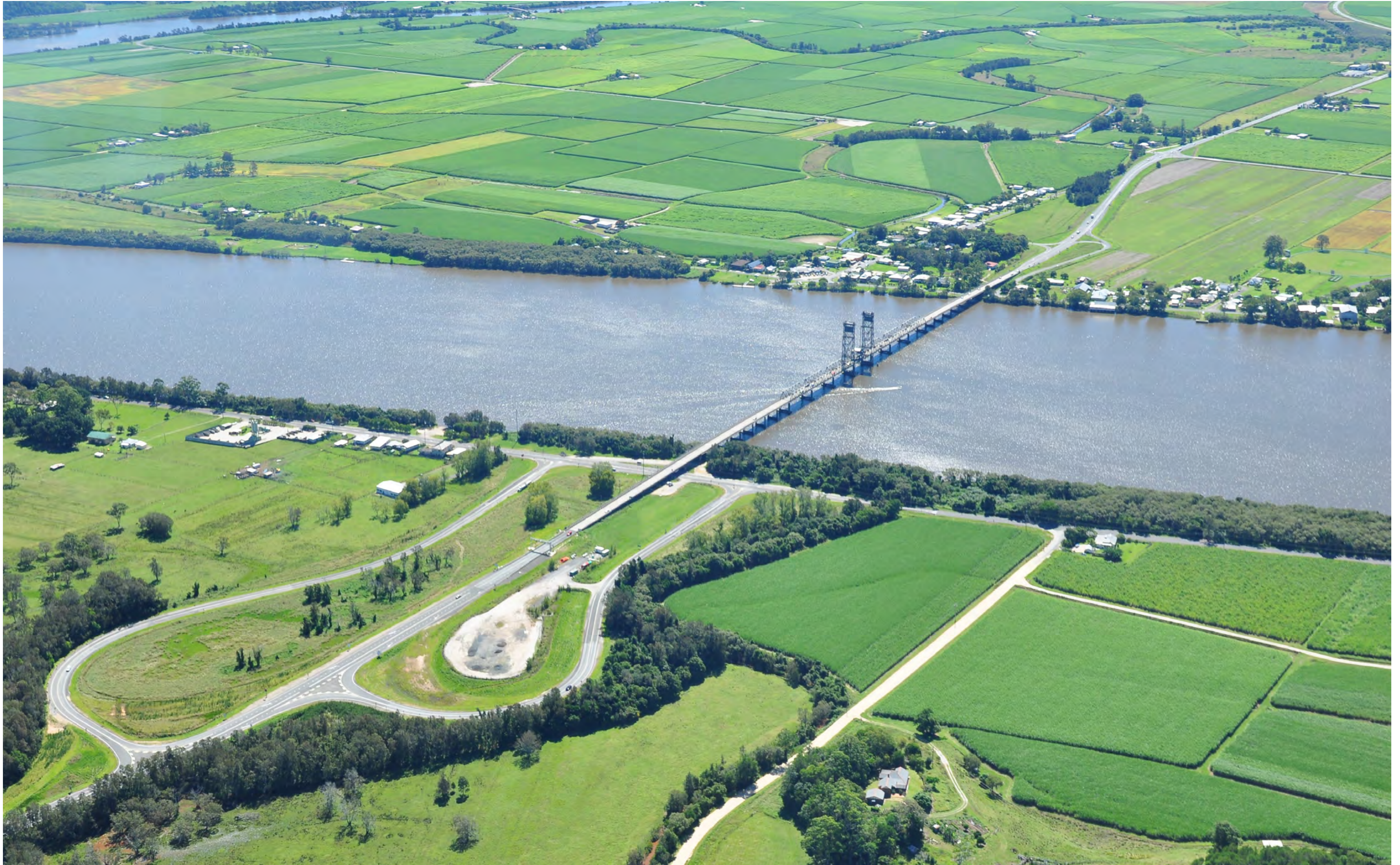
Plate 1-1 Oblique aerial photograph of the existing Harwood Bridge at Harwood crossing the Clarence River looking north west
