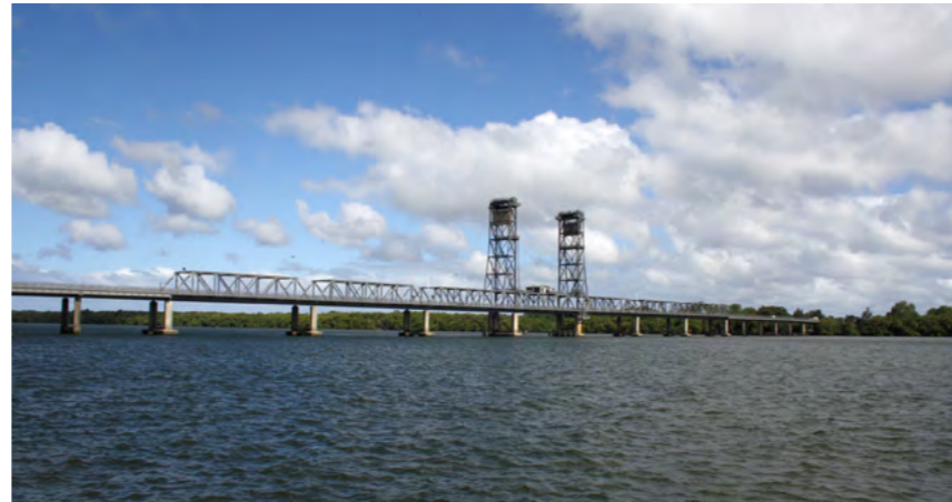
Plate 5-2: Existing Harwood bridge crossing of the Clarence River VP26B
