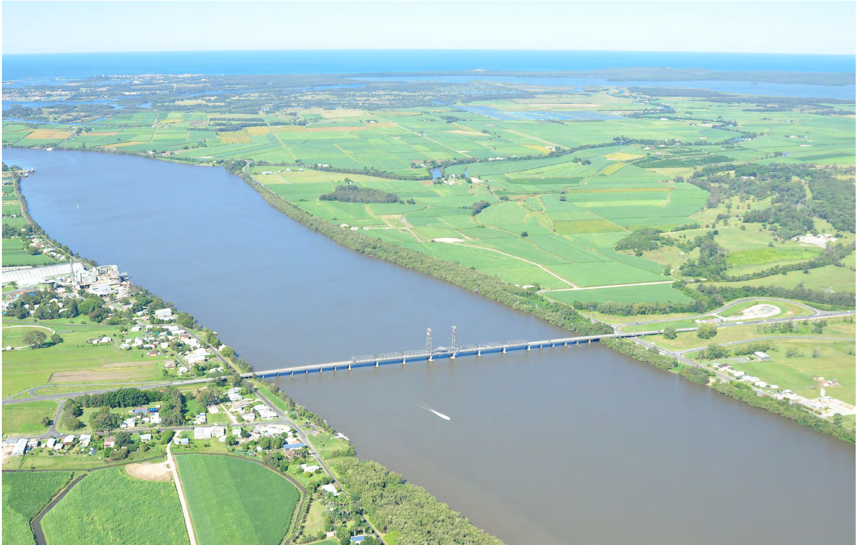
Plate 9-1: Clarence River with the existing Harwood Bridge with the Pacific Ocean in the background. Source: Pacific Complete
