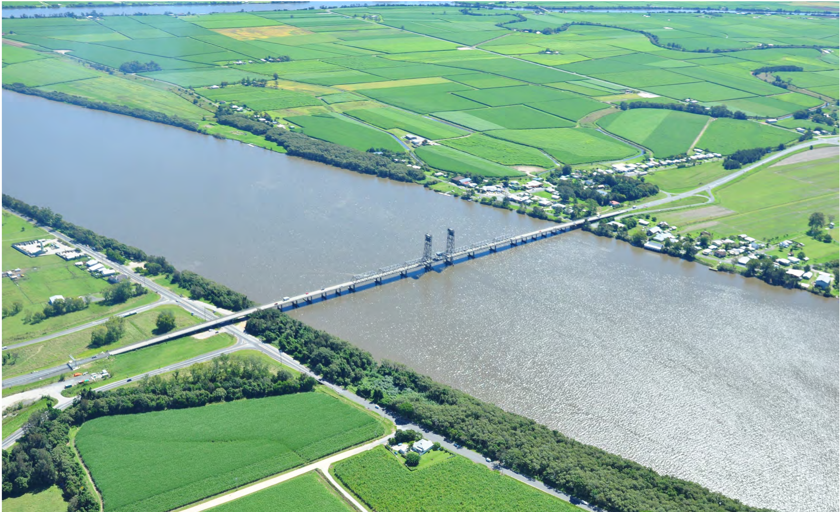
Plate i-1: Oblique aerial photograph of the existing Harwood Bridge at Harwood crossing the Clarence River looking north west
