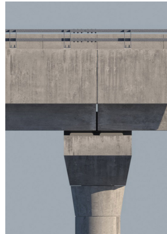
Figure 8.13 Artist impression of bridge headstock Subject to further design
