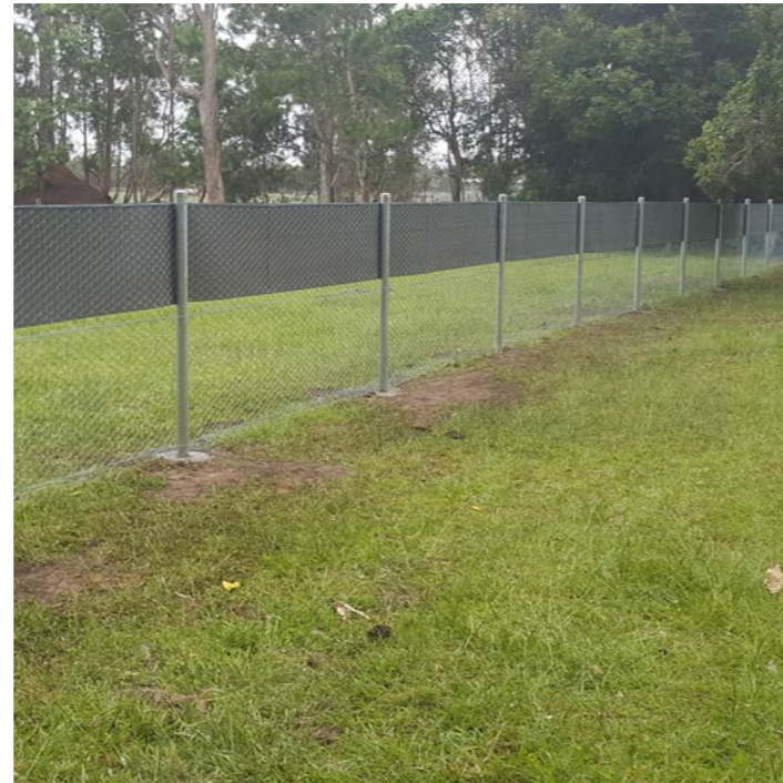
Figure 7.7 Typical fauna fence
