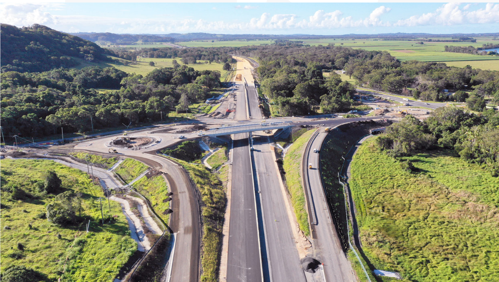
Future Coolgardie interchange looking north, May 2019
