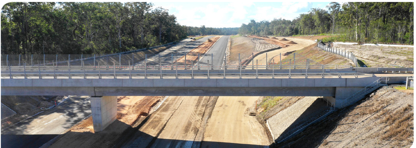
New Bostock Road overpass bridge, Tucabia
