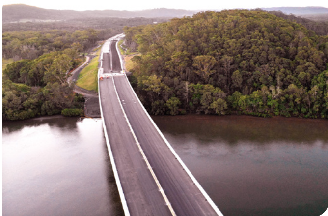
Looking north-west at the new bridge over Richmond River at Broadwater
