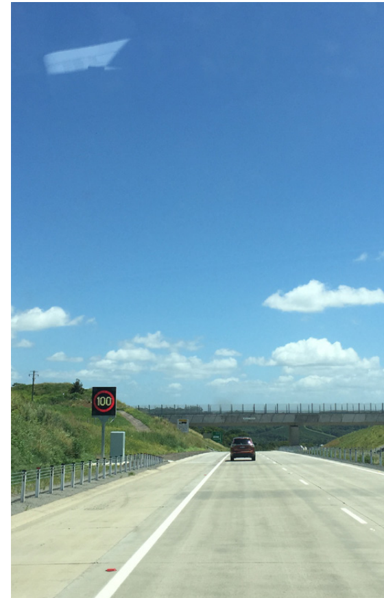
Figure 5.2 Existing Pacific Highway road edge. (Image source: ACJV)
