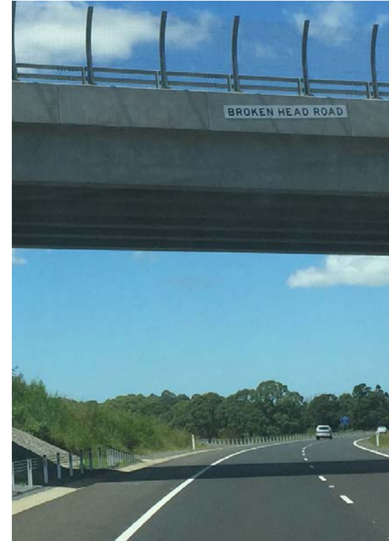
Figure 8.10 Existing bridge parapet and girder
