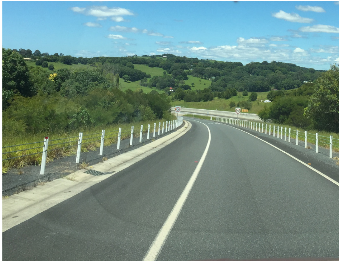
Figure 5.1 Existing Pacific Highway road alignment and character. (Image source:ACJV)
