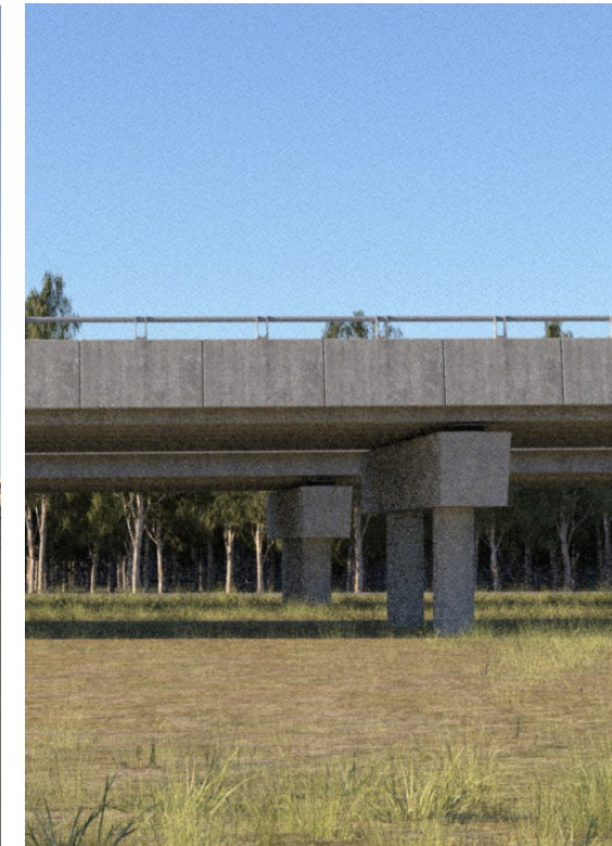
Figure 8.23 Piers and headstock
