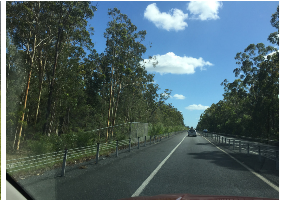
Figure 8.30 Security fencing and wire rope safety barrier
