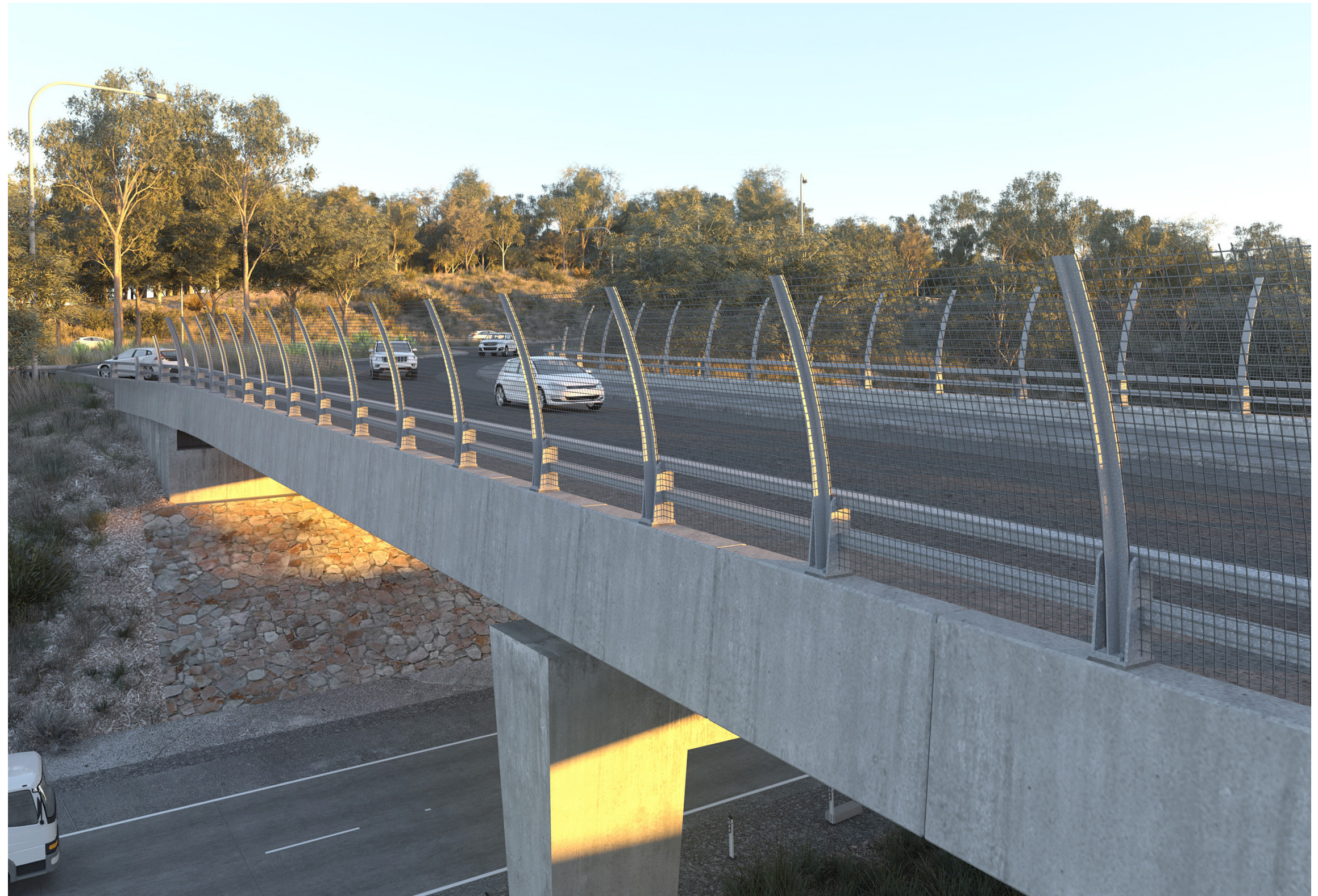
Figure 8.14 Artist impression of bridge at Woodburn Interchange. Landscape shown at full maturity.
