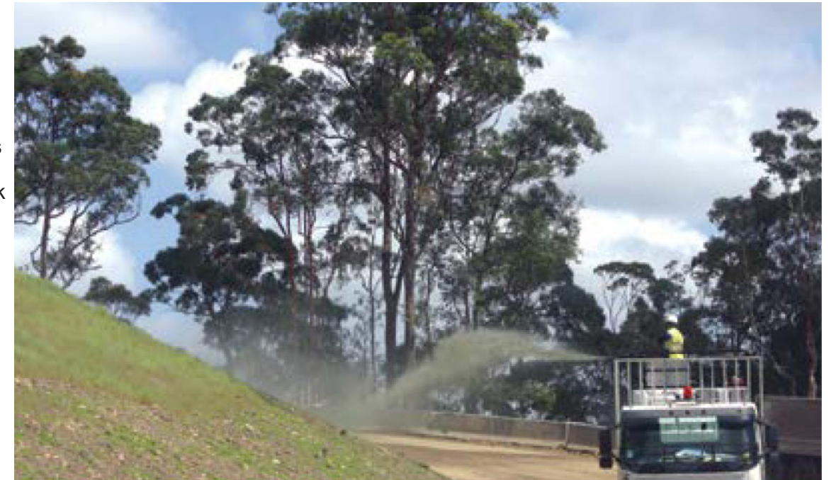
Figure 9.9 Standard Hydroseeding being applied to a batter on the Hunter Expressway.
