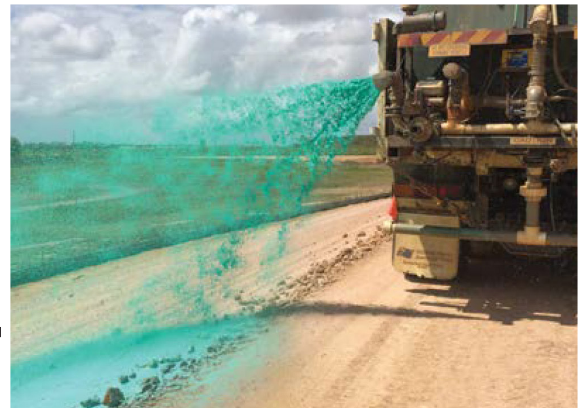
Figure 9.10 Water cart application of a tackifier. (Photo: Vital Chemical Pty Ltd)
