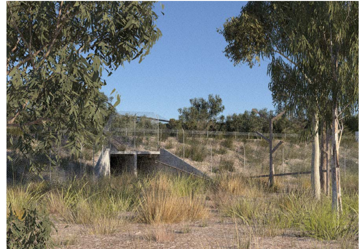
Figure 12.0 Artist impression of fauna culvert with fauna furniture, Landscape shown at full maturity.
