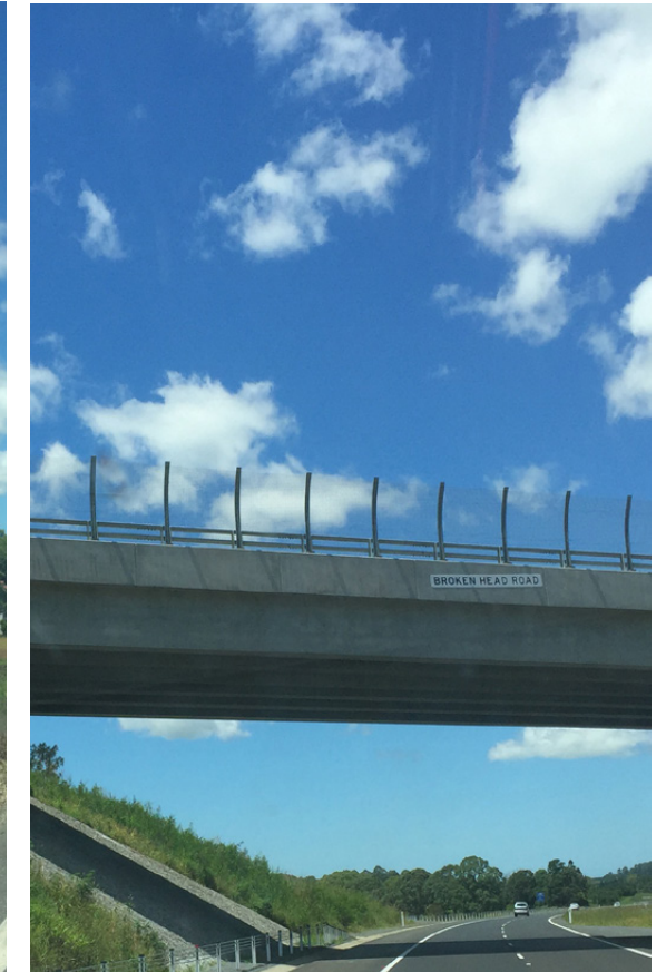
Figure 5.4 Existing landmark of an overpass bridge (Image source:ACJV)
