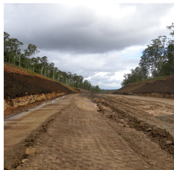
Figure 10.2 Cut batter before roadwork and planting
