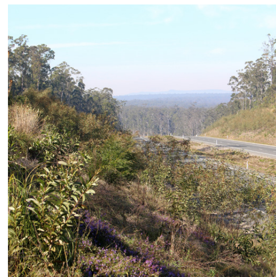
Figure 10.6 Cut batter with established planting
