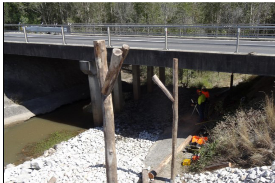
Figure 5.12 Fauna furniture next to underpass bridge Image by Faunacrossings.com.au
