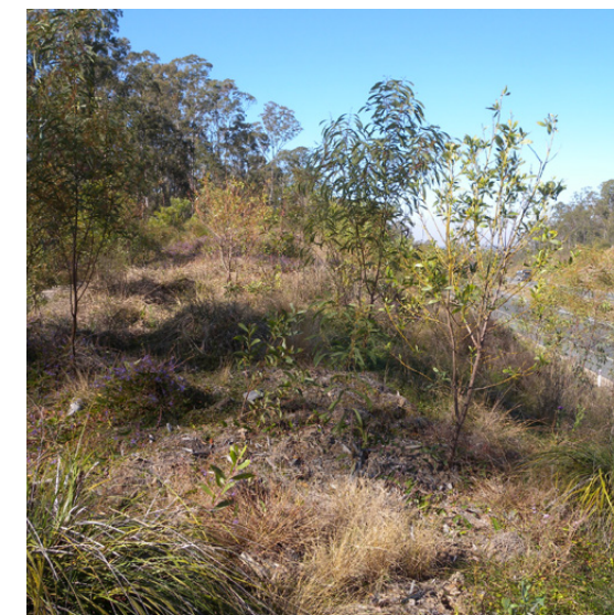
Figure 10.8 Cut batter with mature planting one year after establishment
