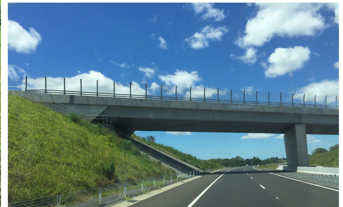
Figure 6.3 Existing bridge, (Image source: ACJV)
