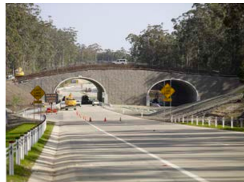
Figure F3: Bonville Koala Bridge September 2008.
