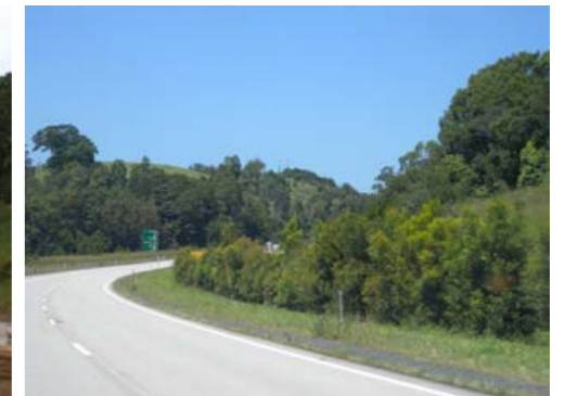
Figure F2: Ballina Bypass January 2015.
