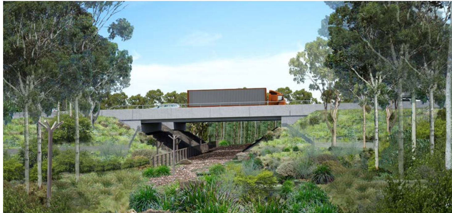
Figure 10: Twin bridges over combined fauna and drainage crossing.
