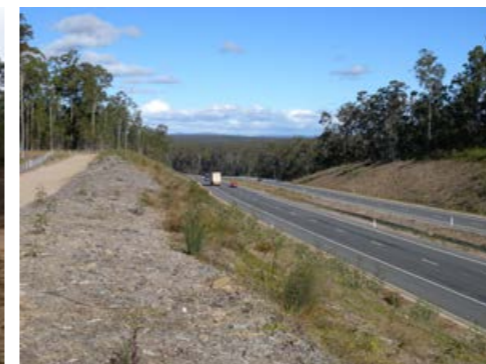
Figure F9: Glenugie upgrade July 2012.
