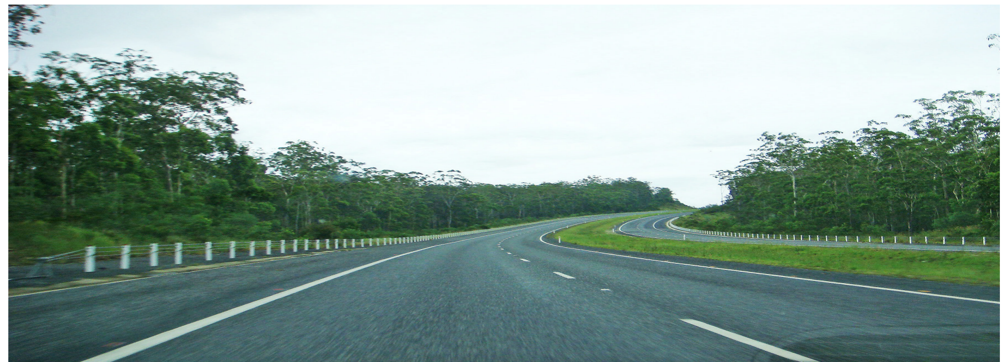
Figure 55: Pacific Highway looking north at Glenugie.
