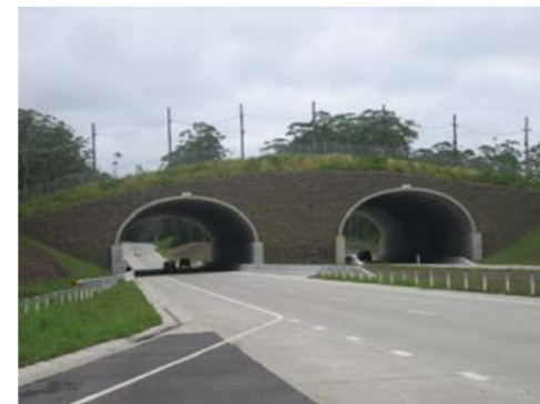
Figure F4: Bonville Koala Bridge February 2009.
