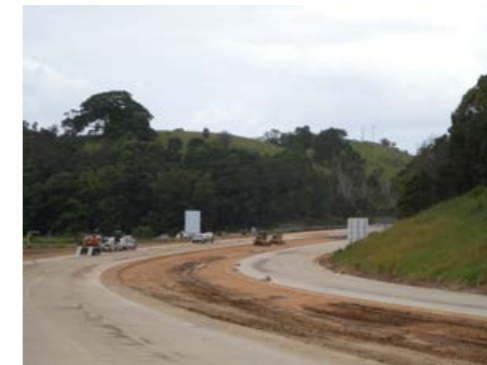
Figure F1: Ballina Bypass February 2011.
