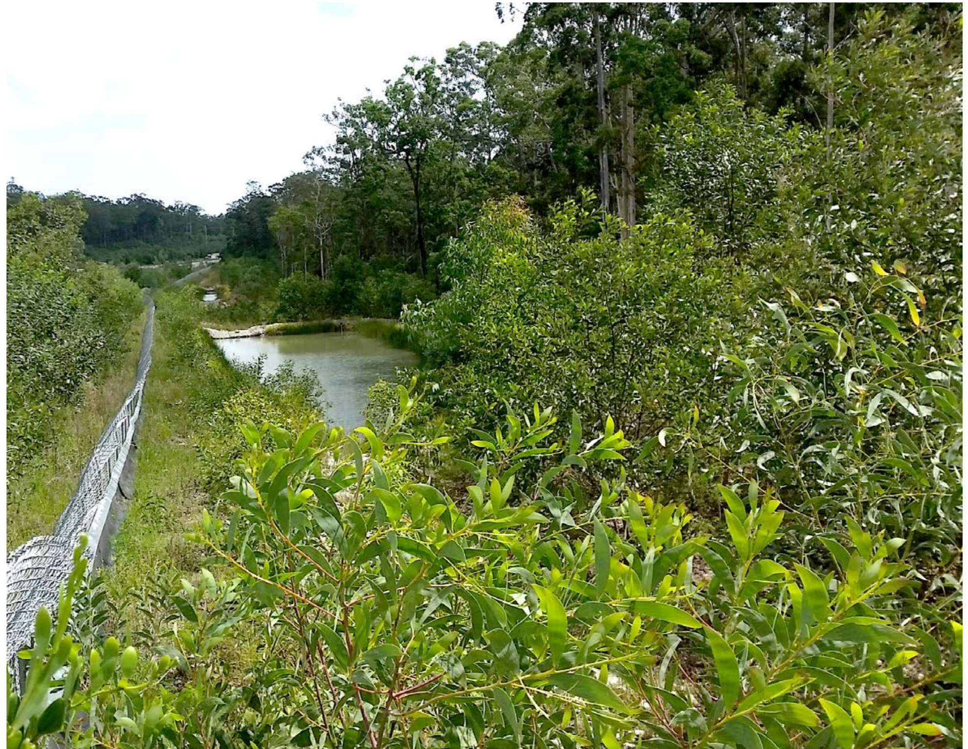
Figure 104: Typical water quality basin on the Pacific Highway at Devils Pulpit with floppy top fauna fencing.
