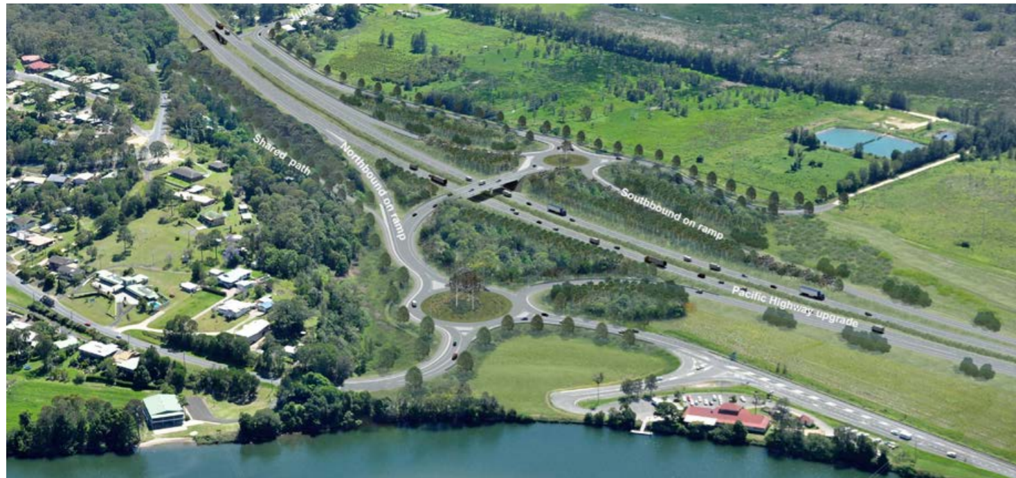
Figure 8: Maclean interchange – aerial view looking north.
