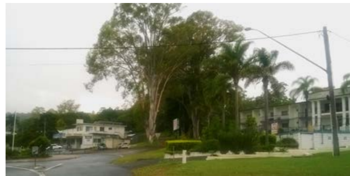
Figure 43: View of Tyndale from existing Pacific Highway.
