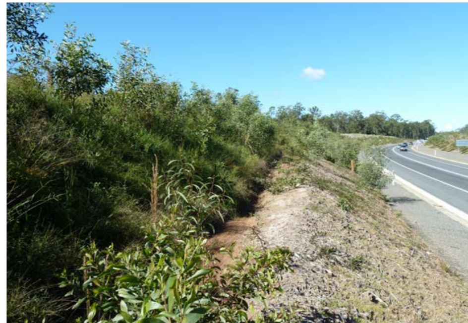
Figure 96: Glenugie batter slope soon after completion showing germination from the soil seedbank.
