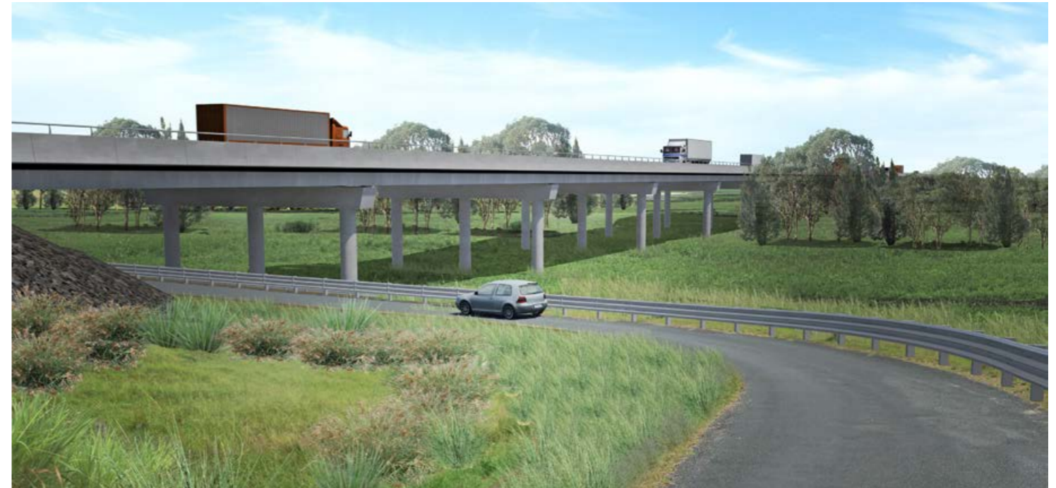
Figure 11: Bridge over Shark Creek.
