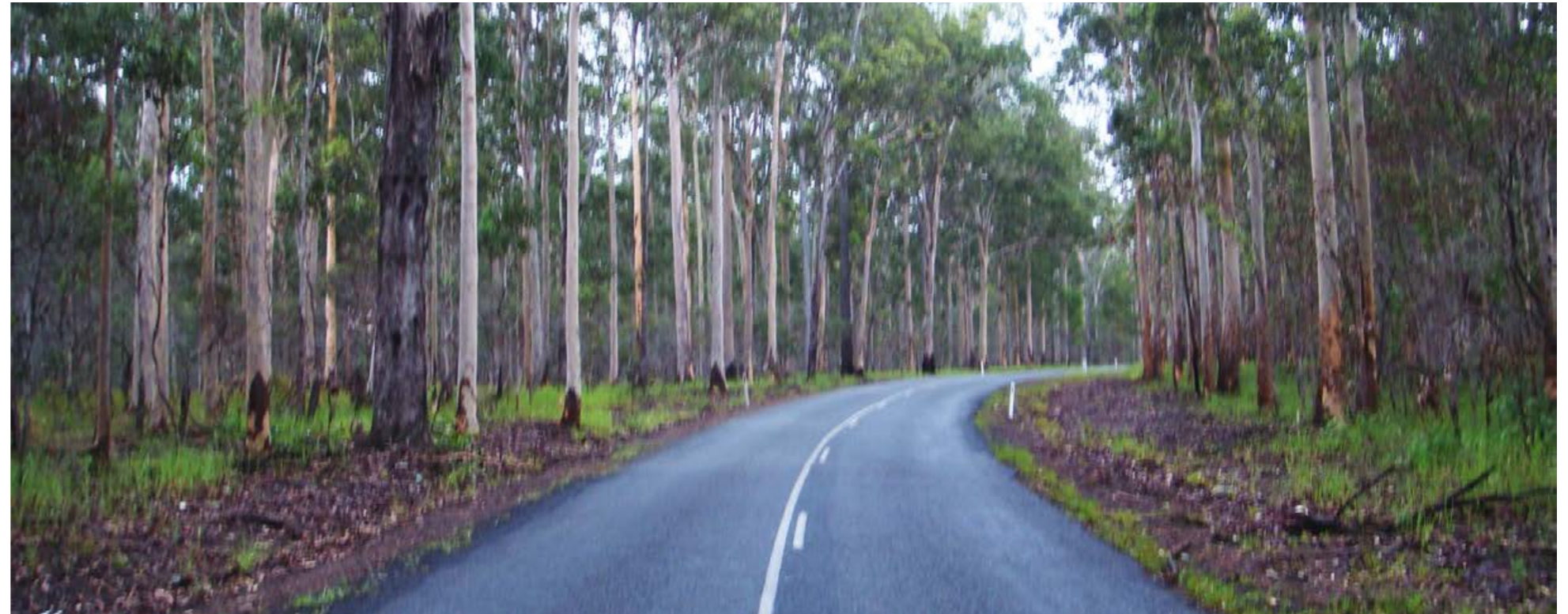
Figure 57: Location of Eight Mile Lane interchange near proposed overbridge.
