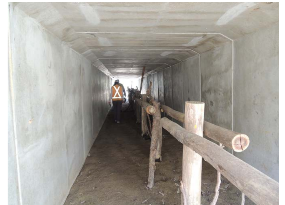
Figure 8-47: Example of fauna furniture inside culvert
