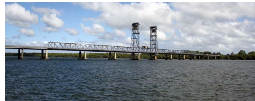
Plate 5-2: Harwood Bridge crossing of the Clarence River
