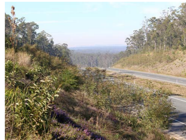
Plate 8-8: Glenugie Upgrade, August 2013
