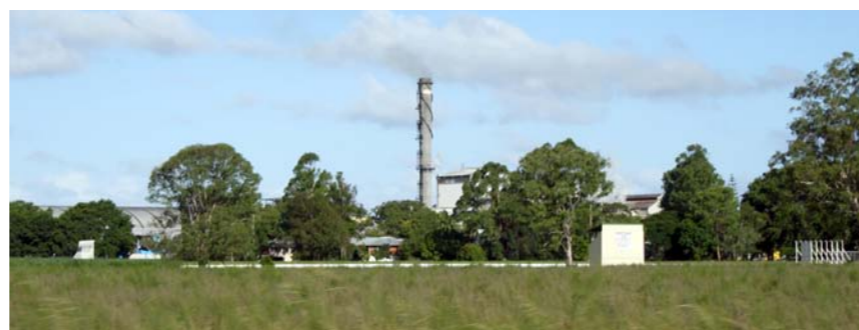
Plate 5-10: Harwood Sugar Mill dominates the skyline at Harwood
