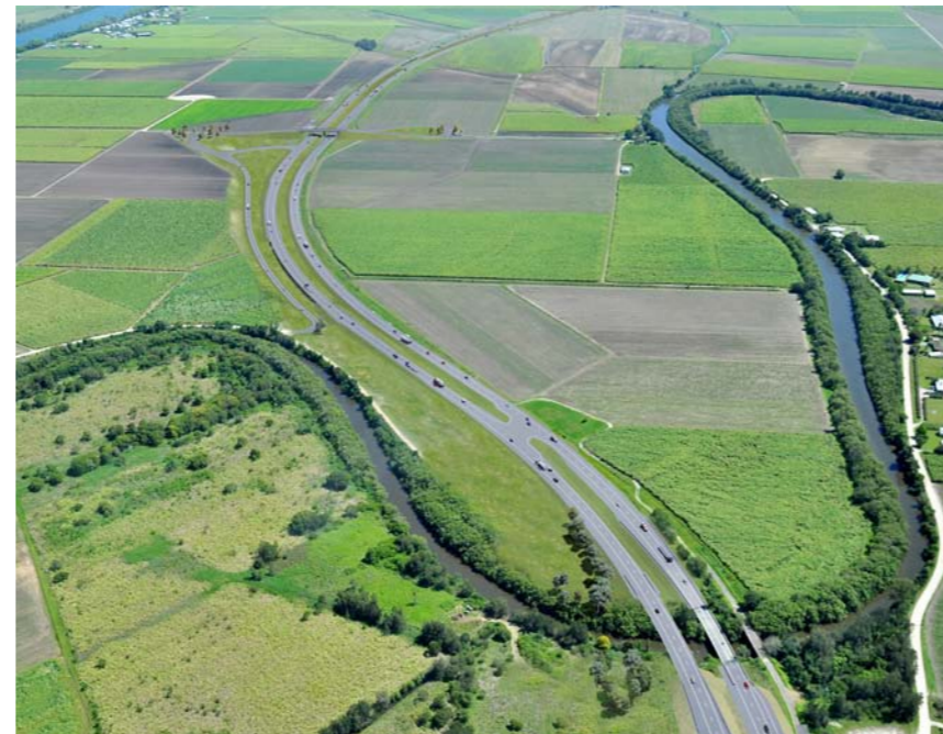
Figure i-1: Artist's impression of highway upgrade through agricultural floodplain on Harwood Island and Chatsworth Island (refer to Chapter 6).
