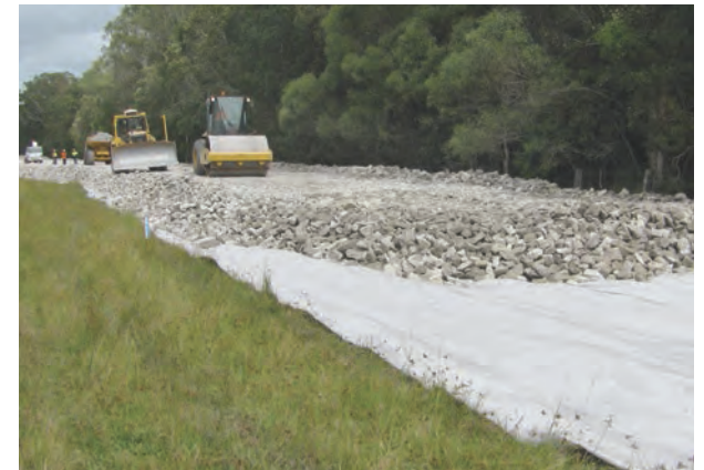
Installing bridging rocks on the floodplain
