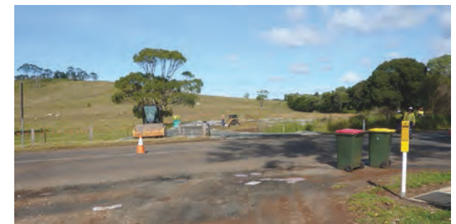
Early work at the Bangalow site compound
