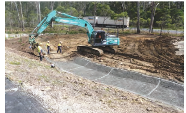
Construction of a concrete drainage structure
