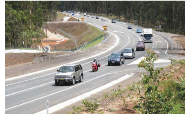
Traffic switch onto a new section of road at Glenugie upgrade
