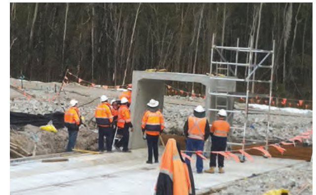
Installing the first culvert for the project
