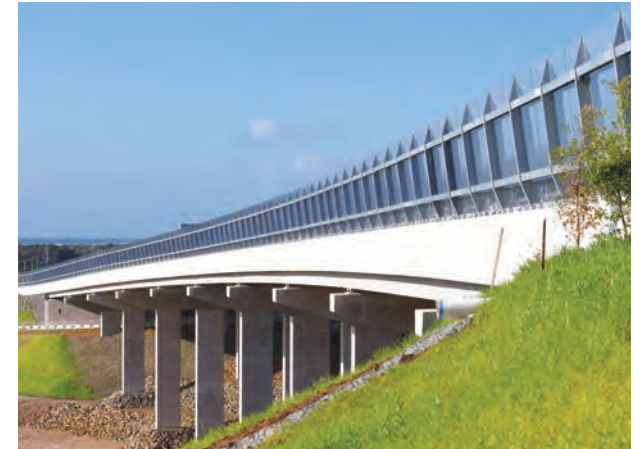
Banora Point upgrade – southern valley viaduct
