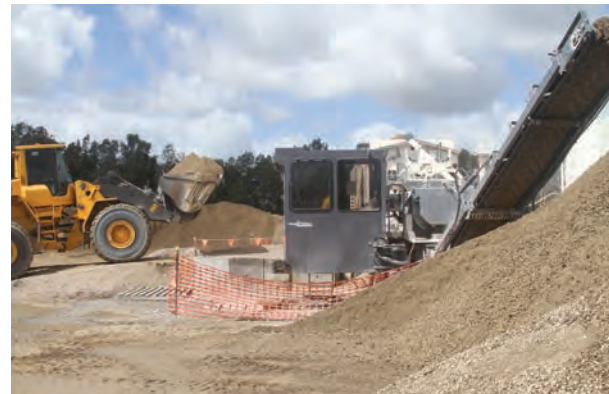
Loading gravel into the batch plant at Farlows Flat
