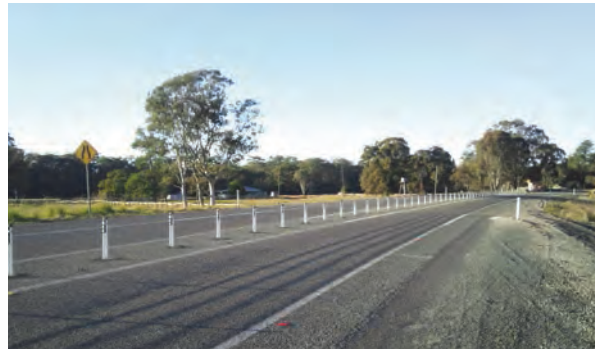
Wire rope installed at Blackadder Creek
