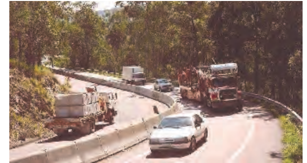
Bulahdelah to Coolongolook project and its dangerous bends before the upgrade program (circa 1990)
