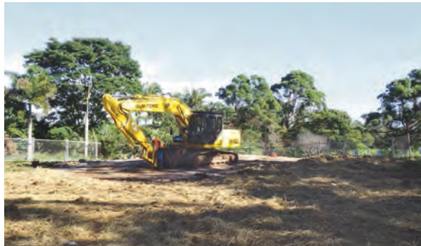
Demolition work at Tintenbar to Ewingsdale
