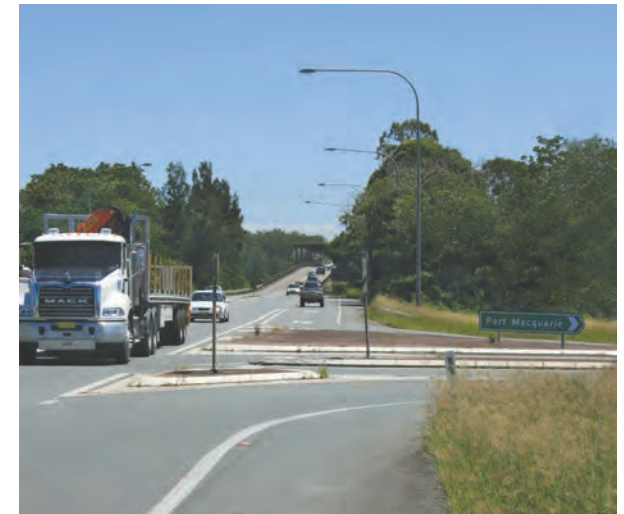
The existing Oxley Highway to Kempsey section
