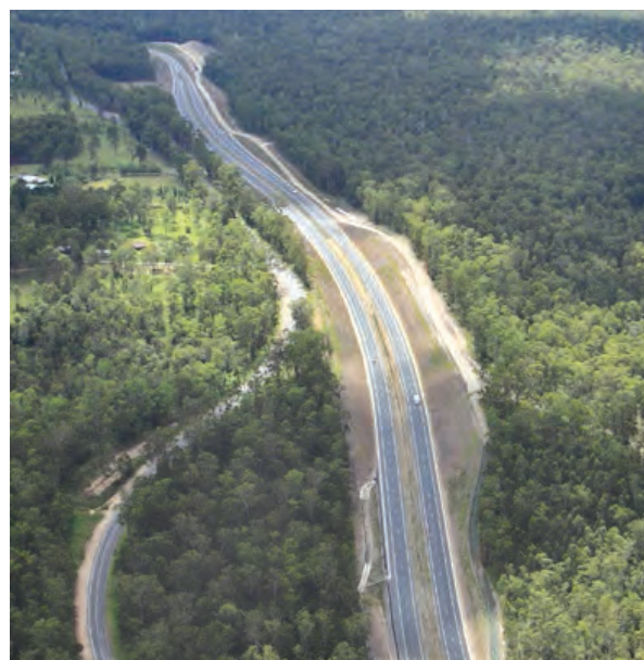
The final section of the Glenugie upgrade is now open to traffic
