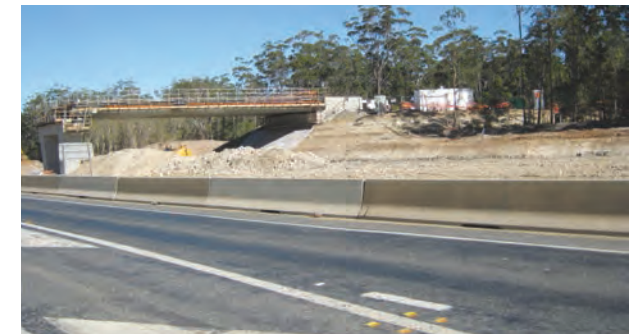
Construction continues on the Arrawarra interchange
