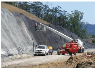
Bulahdelah upgrade – rock bolting work north of Bombah Point bridge
