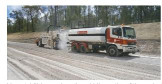
Lime stabilising work on the middle section of the project
