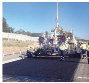
Sapphire to Woolgoolga upgrade - laying of the low noise road surface on the new highway south of Woolgoolga
