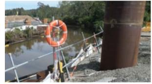
The working platform built to improve safety for workers welding piling casings on the Pimlico to Teven project
