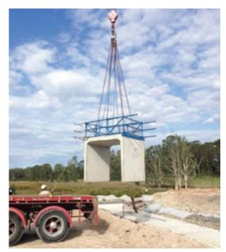
The handrail being used to increase safety for culvert work on the Frederickton to Eungai project
