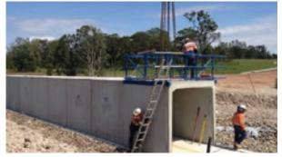
The handrail being used to increase safety for culvert work on the Frederickton to Eungai project
