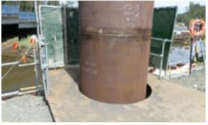
The working platform built to improve safety for workers welding piling casings on the Pimlico to Teven project
