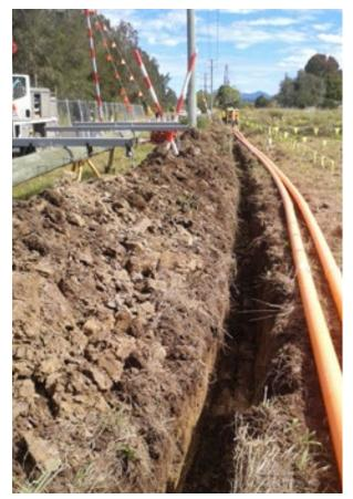
Warrell Creek to Nambucca Heads - Looking west at underground relocation of electrical cables on Nursery Road in preparation for bridgework
