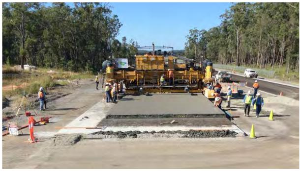
Work in progress to place mainline concrete paving, just north of the Hastings River, Oxley Highway to Kundabung project (March 2016)
