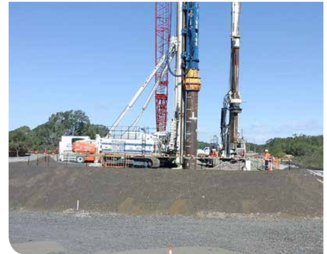
Devils Pulpit to Richmond River, piling for service road (June 2017)
