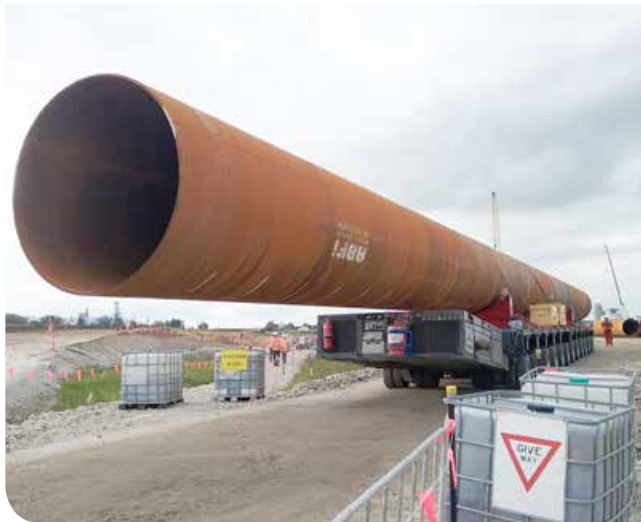
Moving pile casings into place for land piling at Harwood bridge (June 2017)
