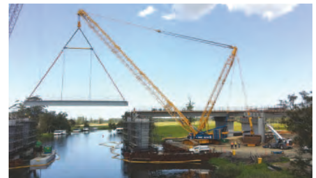
First girder installed over the Myall River at the Bulahdelah upgrade
