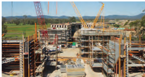
Looking south across the Myall River at the formwork required for the bridges
