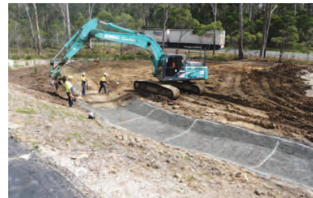
Construction of concrete drainage structure
