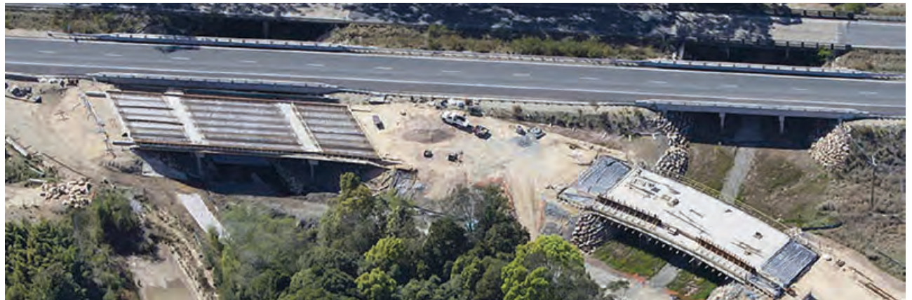
Newly built bridges over the Herons Creek floodway (south) and Herons Creek (north) will form part of a new service road
