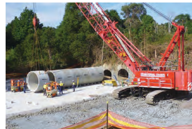
Placement of pipe culvert units at works near Bangalow Road
