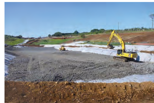
Foundation treatment after excavating silt from the ponds at the old fish farm, Knockrow
