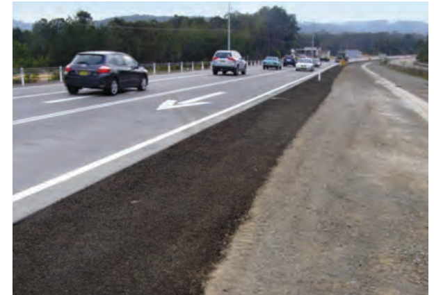
Bulahdelah – traffic being switched onto new northbound carriageway
