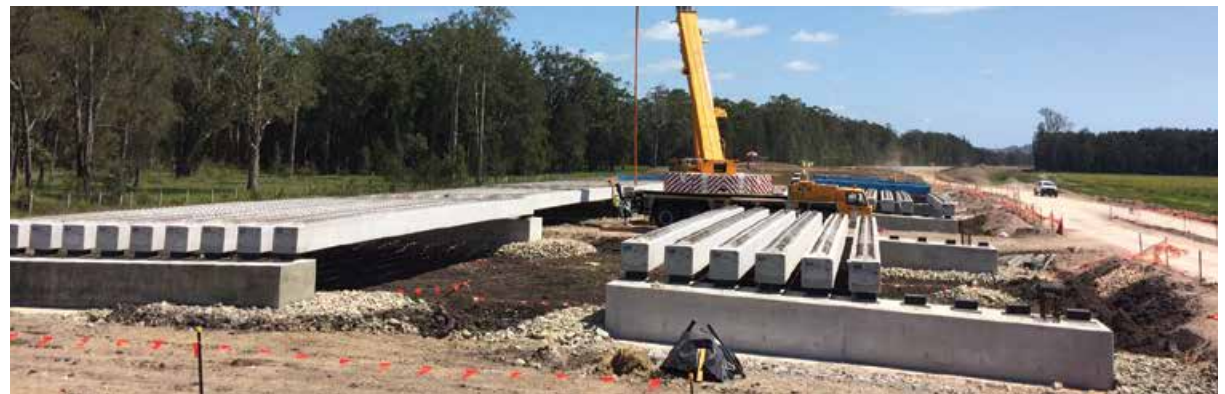
Placing precast bridge planks on a Wilson River floodplain bridge, Oxley Highway to Kundabung project (December 2015)
