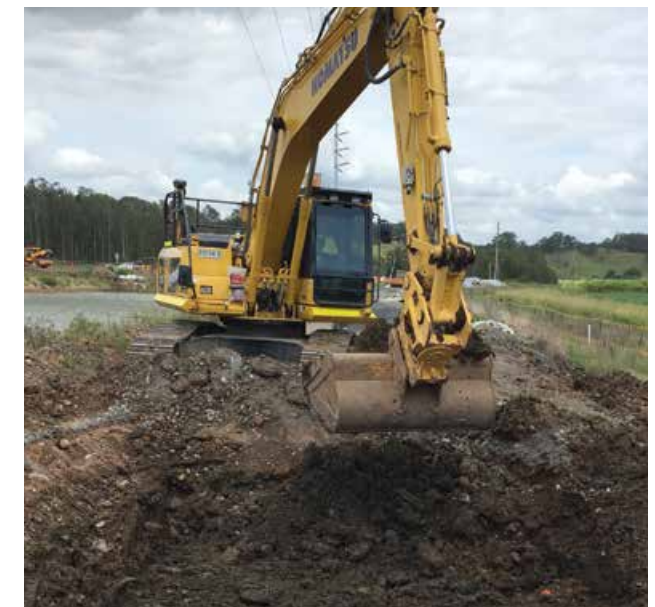
Excavator in operation using electronic control to limit movements
