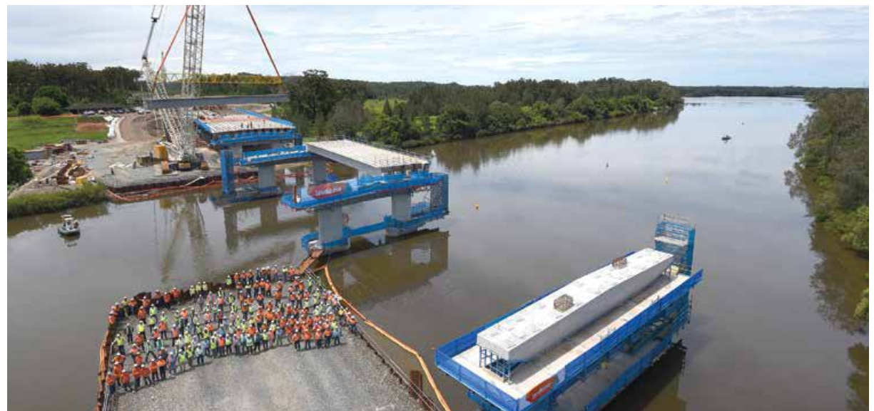
Girder installation on the Wilson River bridge, Oxley Highway to Kundabung project (December 2015)
