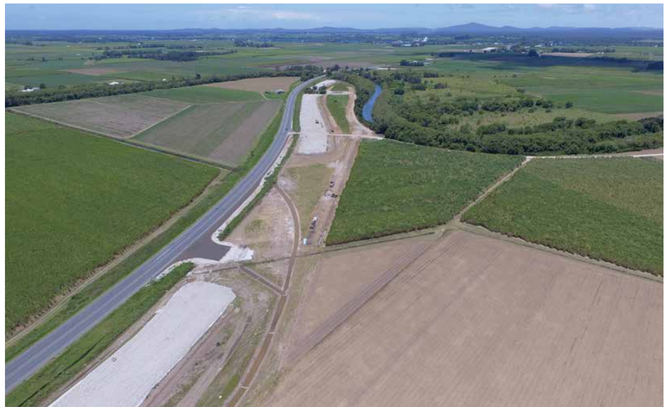
Aerial view of Wave 1 soft soil work on the Woolgoolga to Ballina project (December 2015)
