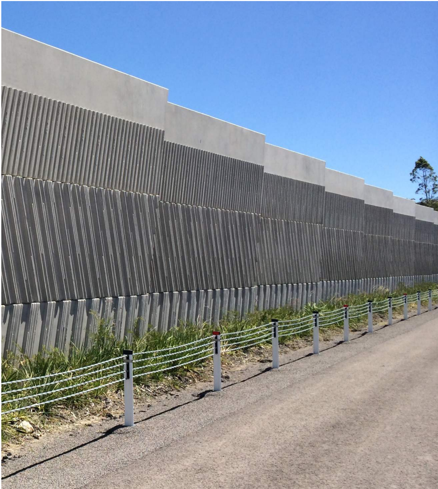
PATTERNED WALLS PROVIDE VISUAL INTEREST THAT CAN RELATE TO CONTEXT AND DISCOURAGE GRAFFITI VANDALISM.
