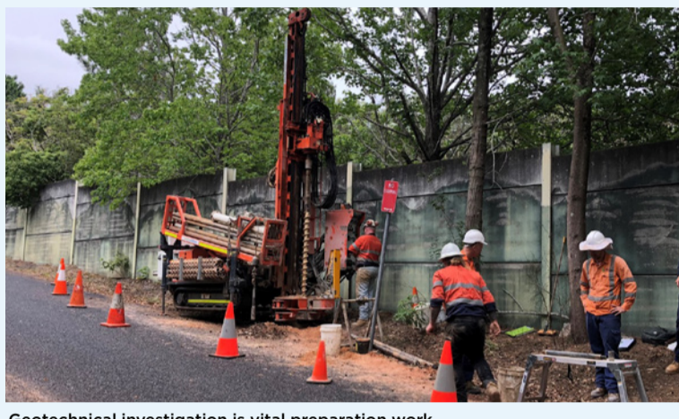
Geotechnical investigation is vital preparation work
