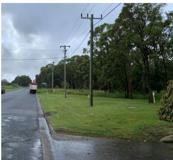
Power relocations will include multiple contractors.
