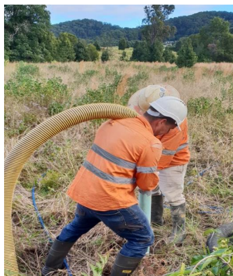
Locating all existing utilities.
