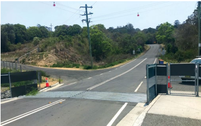
Koala grid on Coolgardie Road (west), installed in December 2019. Koala grids are used in conjunction with fauna fencing to prevent koalas from entering the highway alignment, creating a fully enclosed system.
