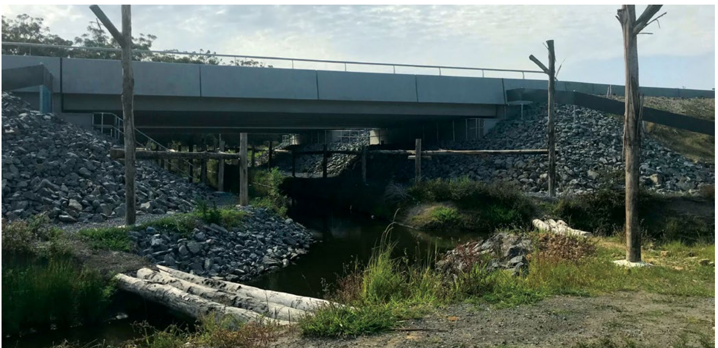
Combined drainage/ fauna bridge underpass on the Pacific Highway south of Wardell Road
