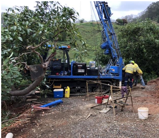
Geotechnical work continues.
