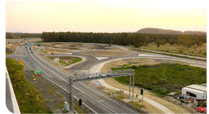
Sunset overlooking the roundabout of the future Yamba interchange
