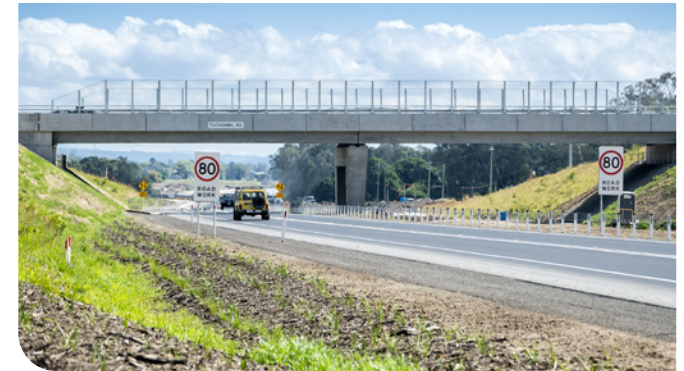
New section of road open to traffic south of Woodburn
