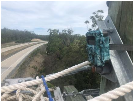
Plate 1: Rope bridges were suspended >10m above the road deck (upper) and supported by poles adjacent to the forest edge. A camera was strapped to the bulkhead at each end of the bridge (lower left). Black core-flute was cable tied to the underside of the rope ladder at each end during year 1 to reduce the incidence of false-triggering caused by traffic (lower right).
