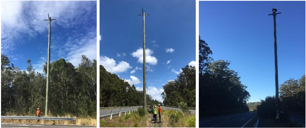
Plate 2: Glide poles stood 19m to 20m above road level and featured perpendicular and parallel-to-road cross arms. GP1 (left) was positioned adjacent roadside forest habitat on the eastern edge of the Solitary Island Way, approximately 50m from the rope bridge at chainage 1800 (RB1). GP2 (mid) and GP3 (right) were positioned within the highway median at Halfway Creek area (chainage 16060 & 16430).
