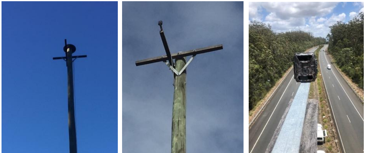
Plate 3: GP3 featured a predator shield above the pole top (left). Cameras were mounted on a flat metal bar and projected ~150mm beyond the end of the parallel glide arm to capture glider activity (mid & right).
