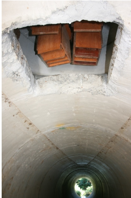
Plate 3.13 Recessed Chamber with Bat Boxes (Source: V. Silver)
