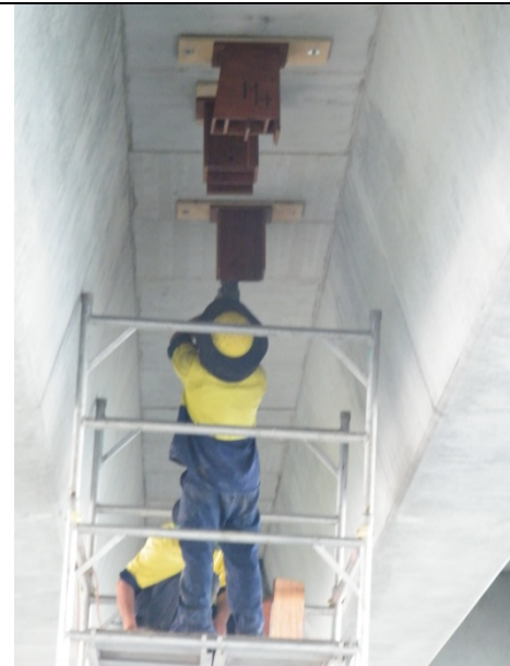
Plate 3.8 Installation of bat boxes beneath Mororo Bridge (Source: D. Andrighetto)
