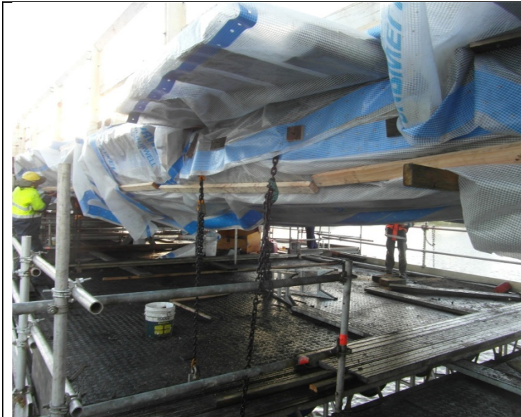
Plate 3.5 Exclusion Option – Plastic wrap bridge (Source: A. Lloyd)
