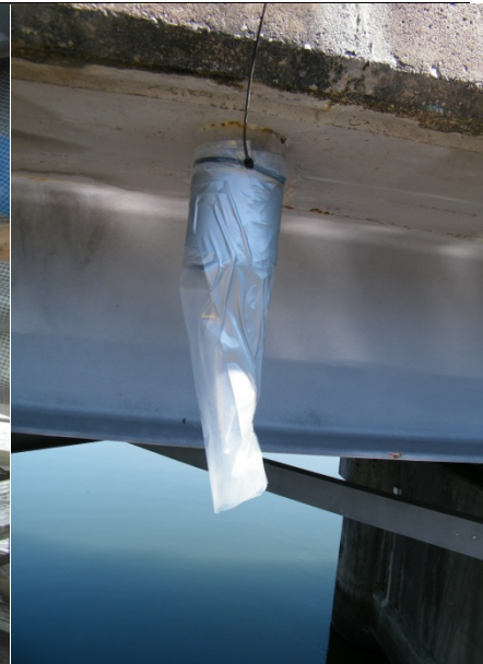
Plate 3.6 Exclusion - Plastic over scuppers (Source: D. Andrighetto)
