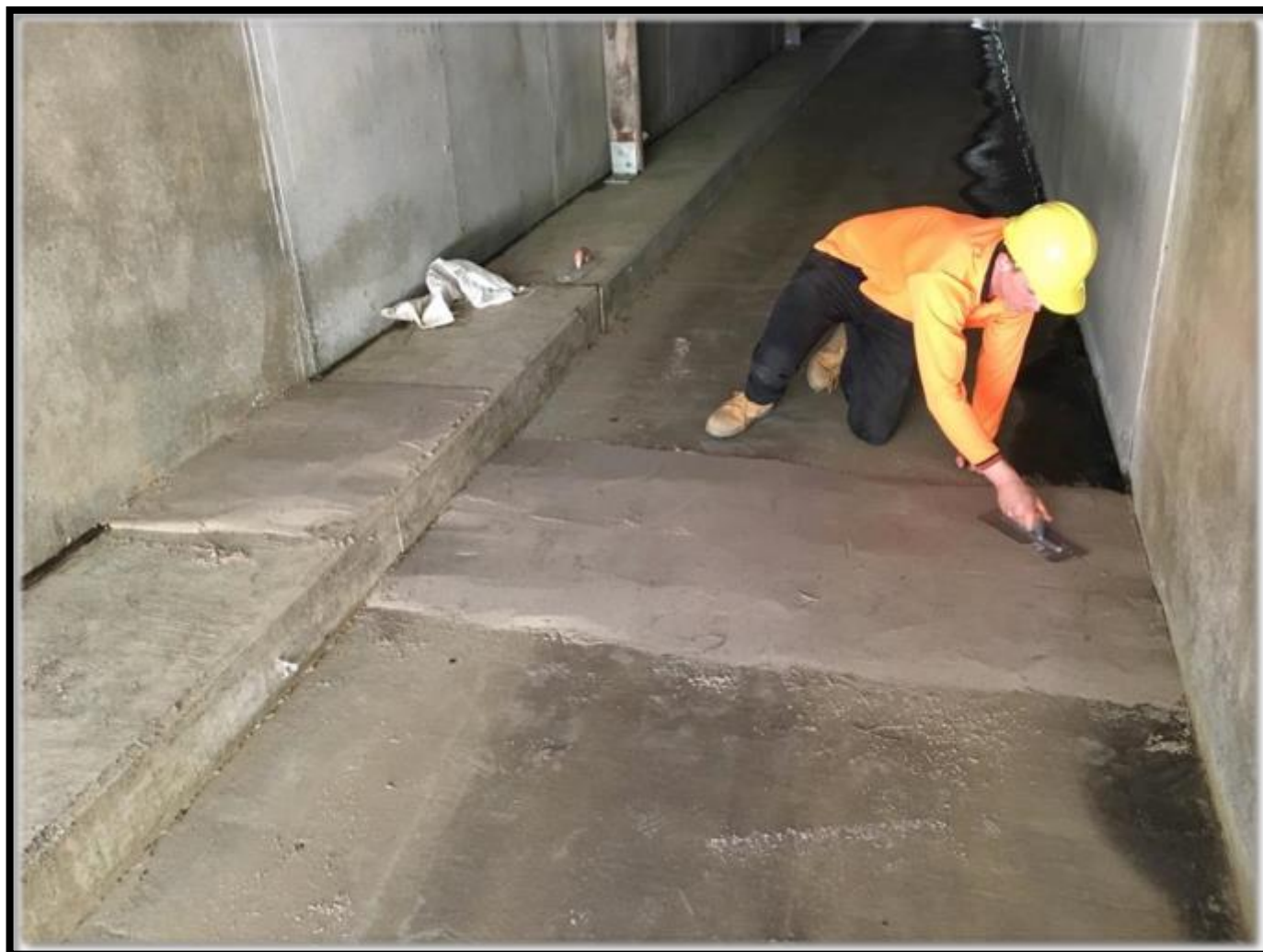
Plate 2. Sand pad being installed in a fauna underpass (Site 3) on the WC2NH upgrade.
